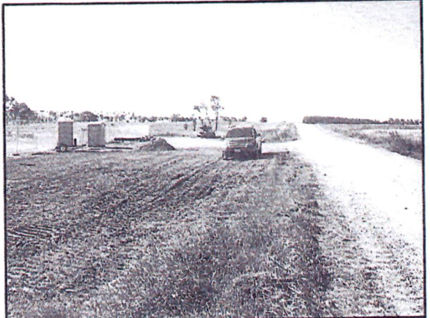
LOOKING SOUTH ON EAST SIDE OF ROAD
