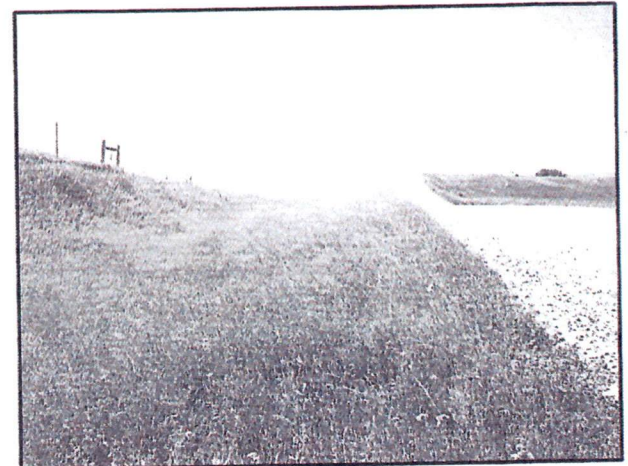
LOOKING SOUTH ON EAST SIDE OF ROAD
