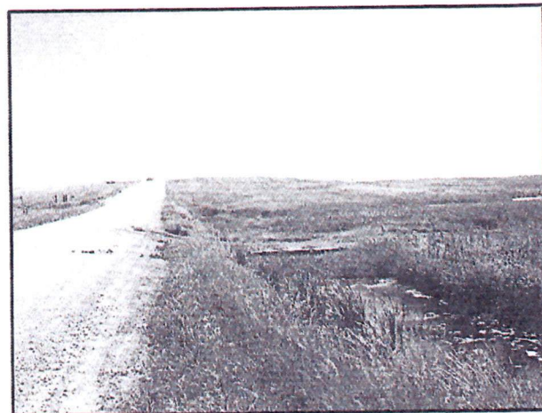
LOOKING SOUTH ON WEST SIDE OF ROAD
