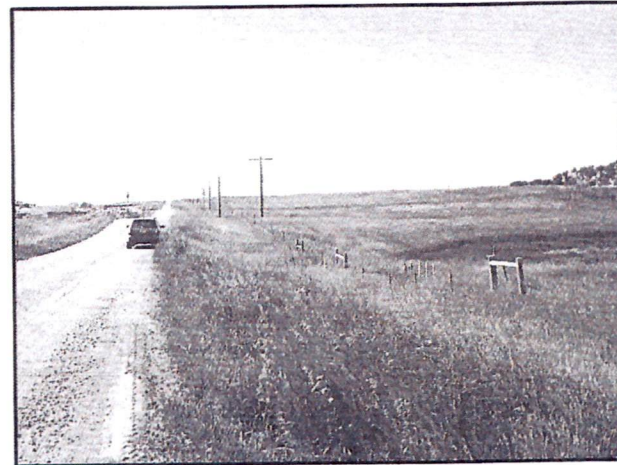
LOOKING SOUTH ON WEST SIDE OF ROAD
