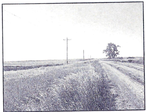
LOOKING SOUTH ON EAST SIDE OF ROAD
