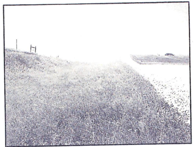
LOOKING SOUTH ON EAST SIDE OF ROAD
