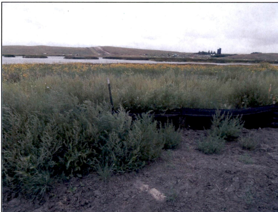
Figure 8. Photo taken looking west along ROW from west side of the Little Knife River. Silt fence borders the location of the bore pit work area appropriately set back from wetland.
