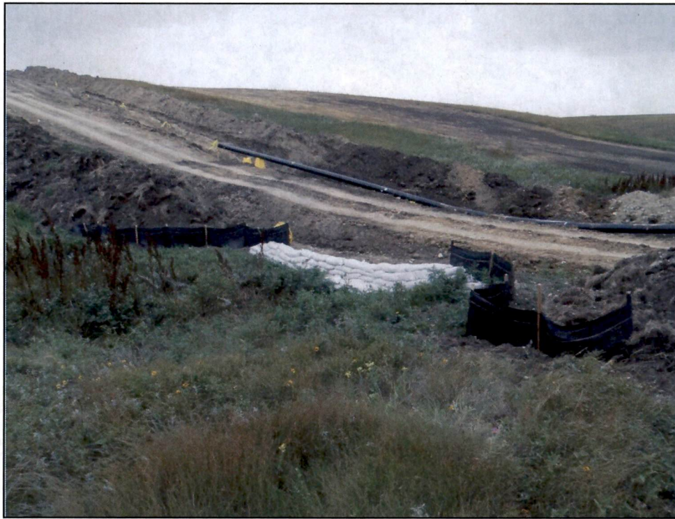
Figure 5. Typical flume pipe crossing of an ephemeral drainage.
