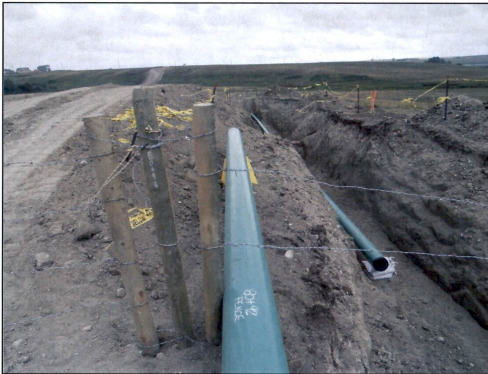
Figure 3. Typical fence line and foreign pipeline crossing.
