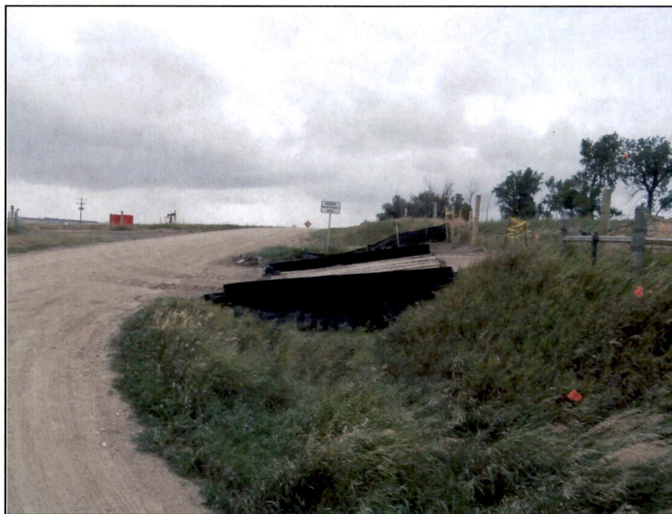
Figure 4. Additional example of road ditch crossing in ROW for vehicles and equipment.
