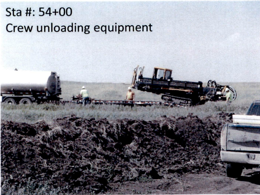
Sta #: 54+00 Crew staging equipment for 80 th Ave bore
