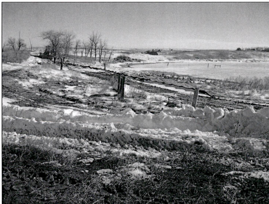
Figure 6. USFWS easement wetland avoided within native grasslands. The easement wetland will be crossed using HDD. A travel corridor is established around the wetland which is protected by silt fence and straw bales.
