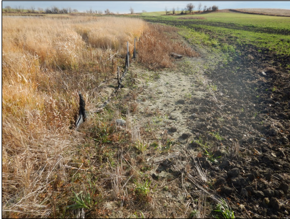
Photo 7. Temporary impacts to wetland edge. Remnants of sediment control features that prevented soil deposition into wetland during construction. Wetland species are reestablishing along the edge with no apparent permanent impacts.
