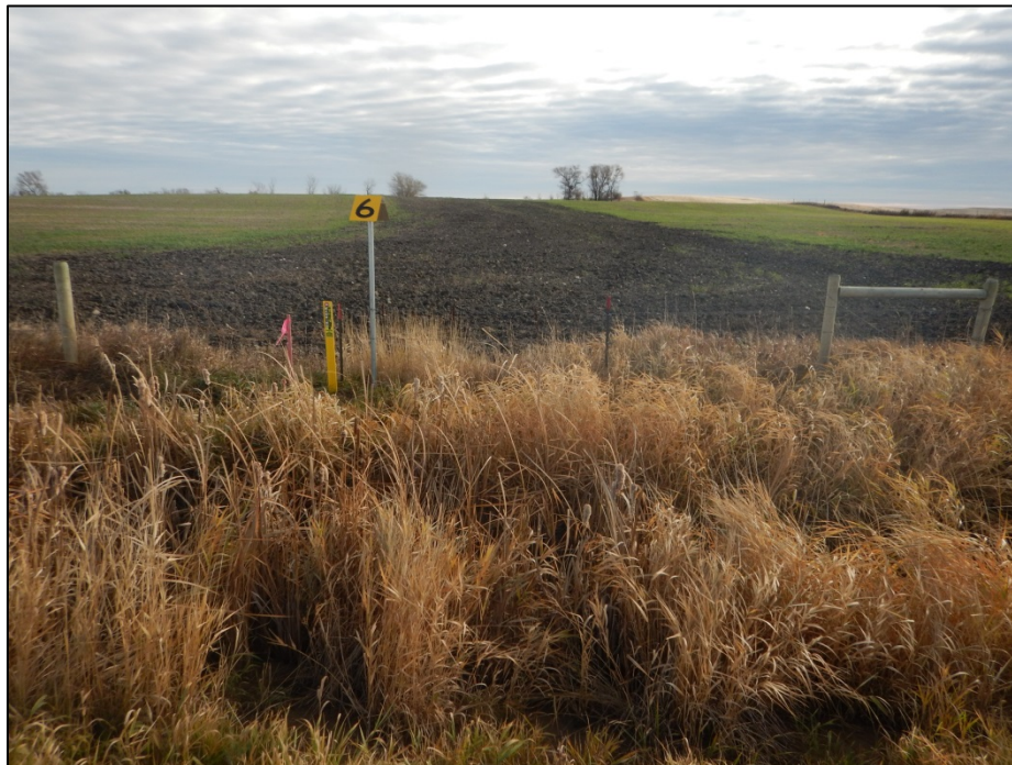
Photo 6. ROW in cultivated agricultural field ROW was disked by landowner or Plains to smooth the reclaimed ROW soils before fall freeze.
