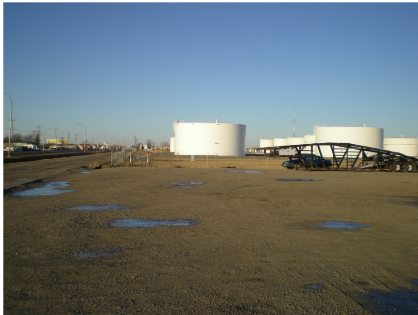
North terminus and Main Ave. road bore workspace
