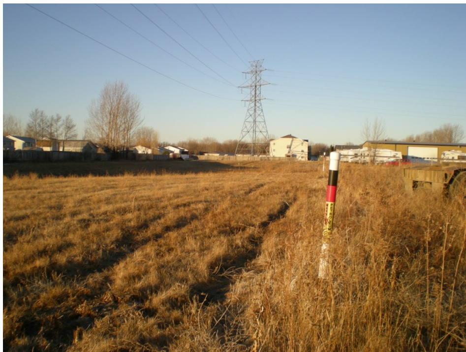
Pipeline marker near east terminus
