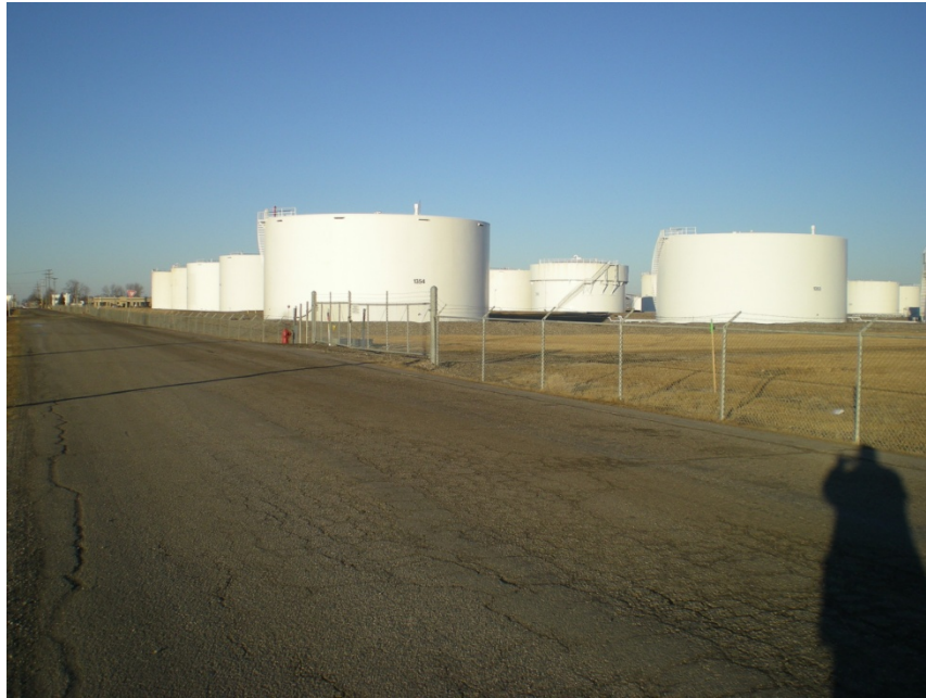
North terminus and tanks
