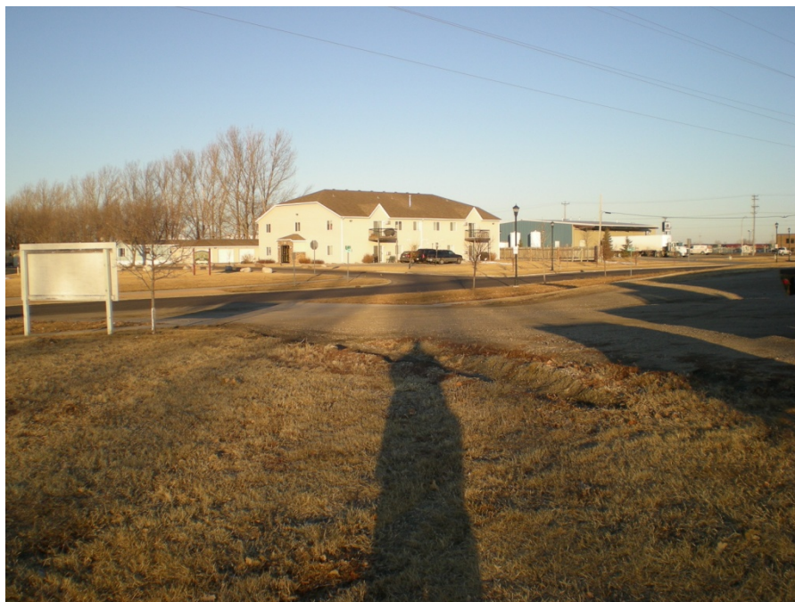
17 th Street road bore looking north
