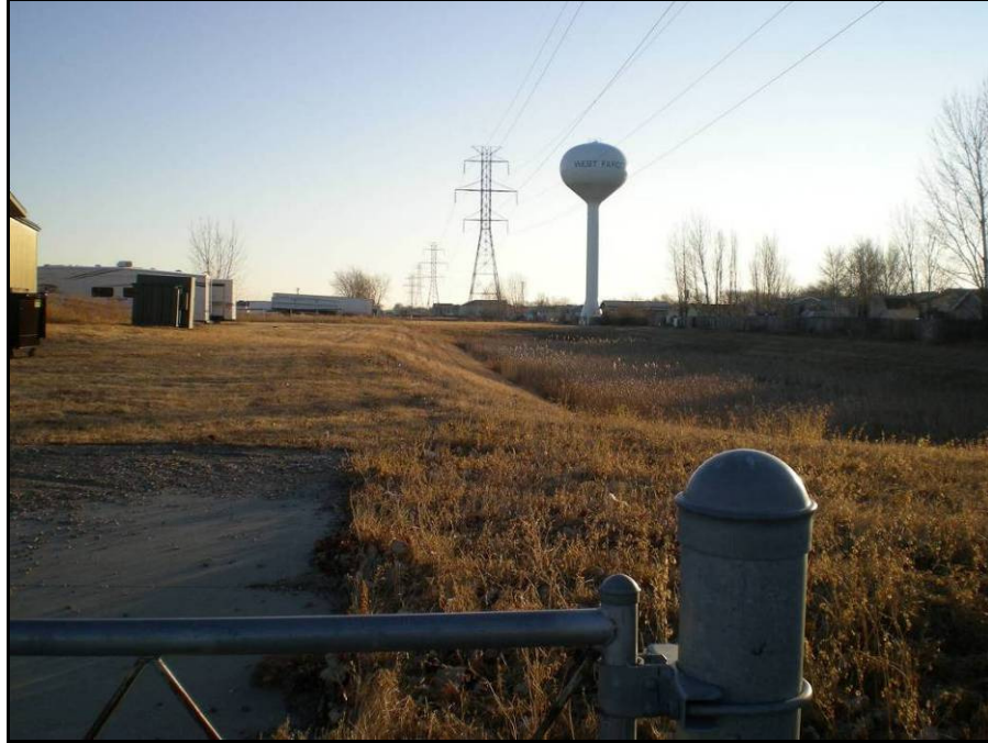
Figure 4. Overview of eastern end of project area, facing east.
