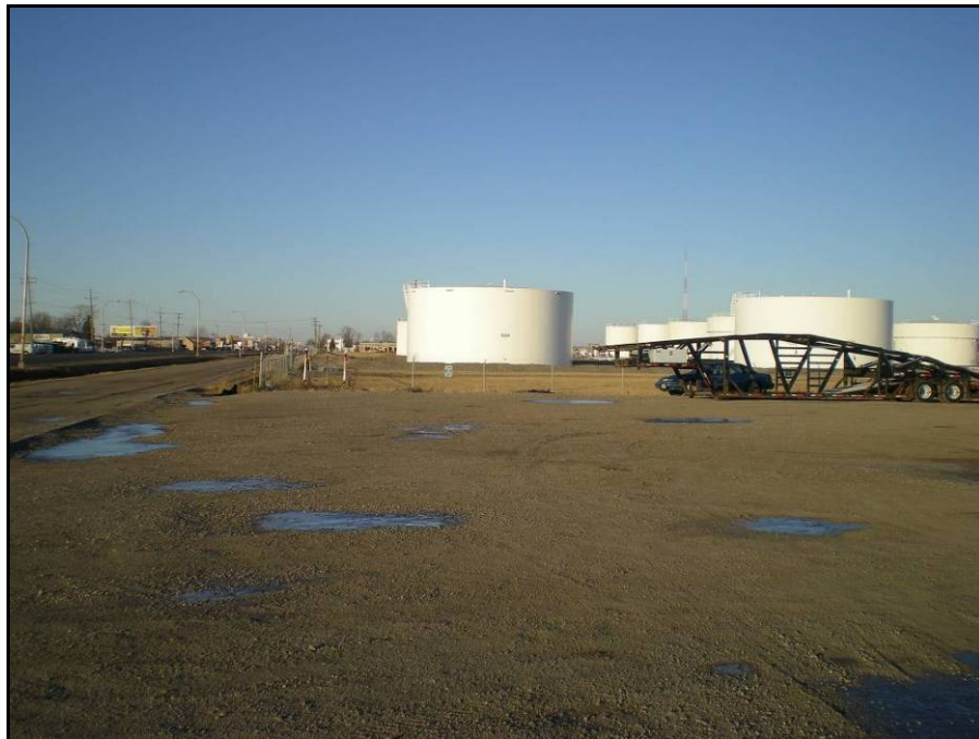
Figure 9. View of corridor at the northern terminus with the terminal storage tanks in the background, facing west.
