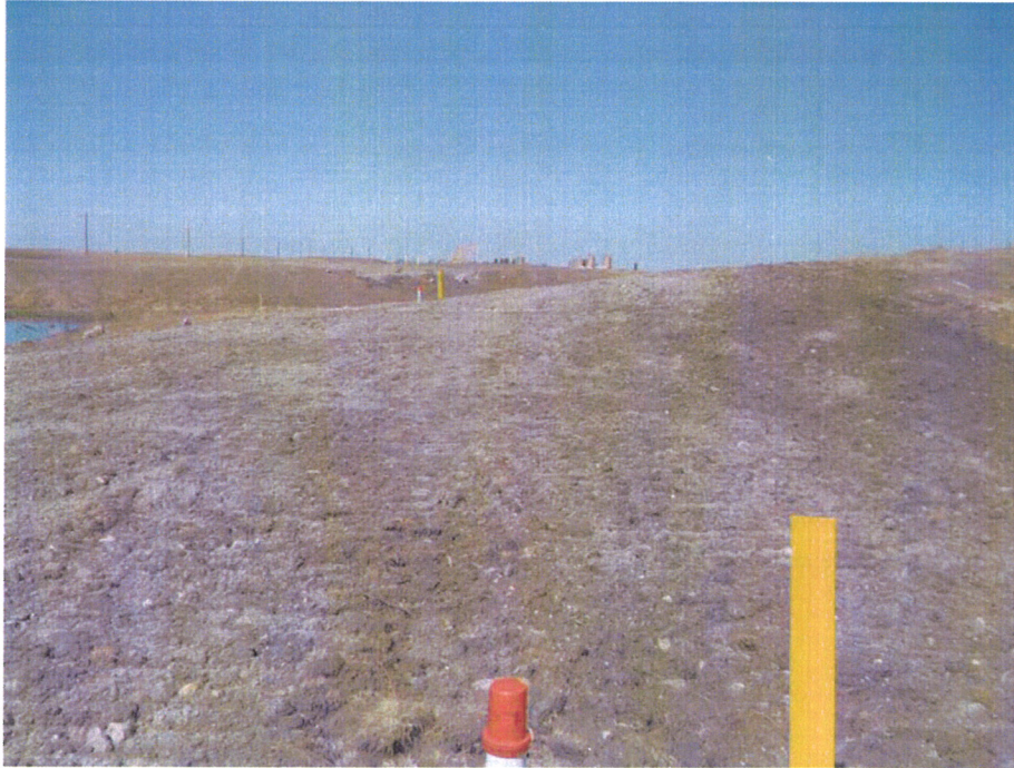
Photo 2 Pipeline loop no vegetation
