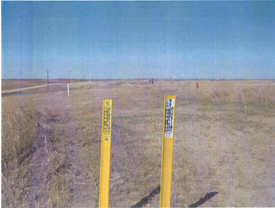
Photo 4 Pipeline loop partial vegetation
