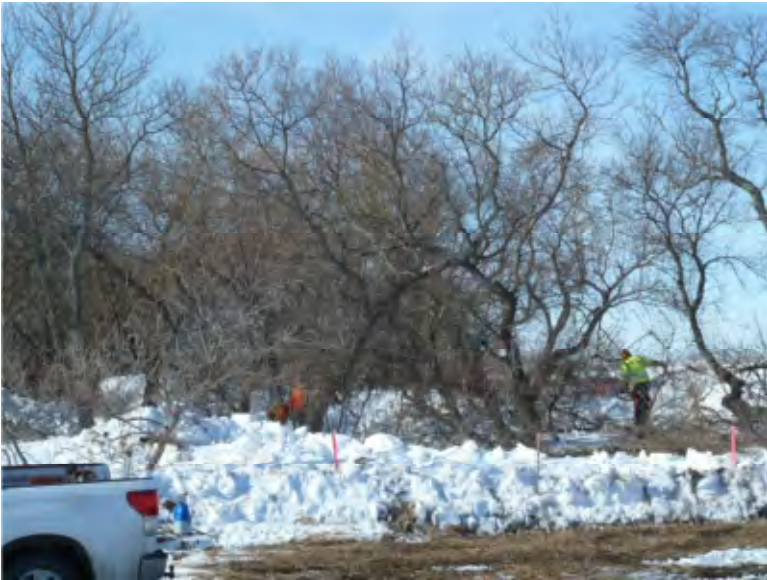
Crews Cutting the Larger Trees - West Site
