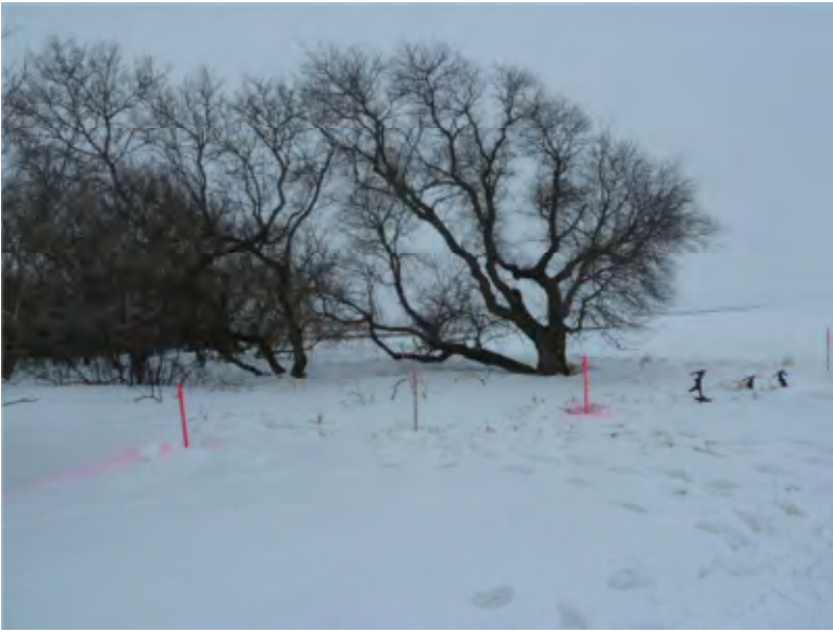
New Alignment Staked – Boxelder Trees, Looking West
