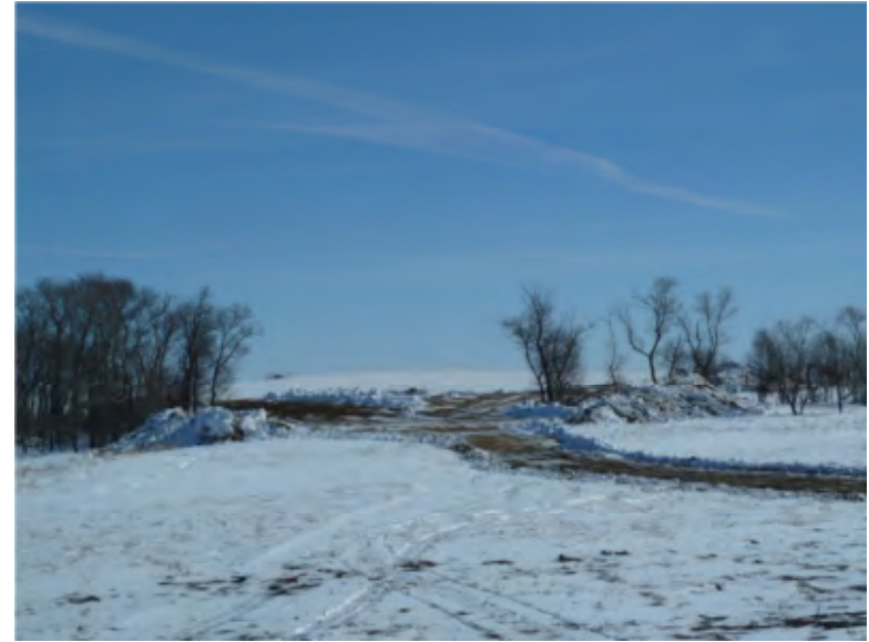
The New Alignment Looking East
