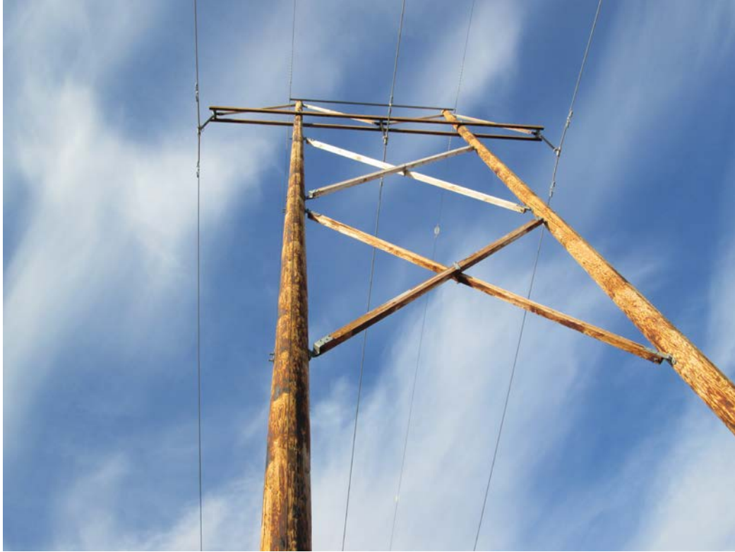
Above: Photo 13 (Structure 553) – Typical double pole structure. Bird diverters along line.
