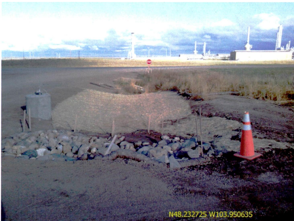
Figure 6. Straw wattles, rip-rap, erosion blankets and silt fencing used to stabilize soils in and around culvert drainage leading into highway ROW ditch.
