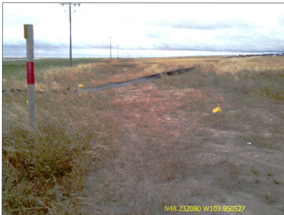
Figure 2. Photo of silt fence and cover crop south of Site. Silt fence in need of minor maintenance but was still working effectively. TIC committed to repairing it immediately.
