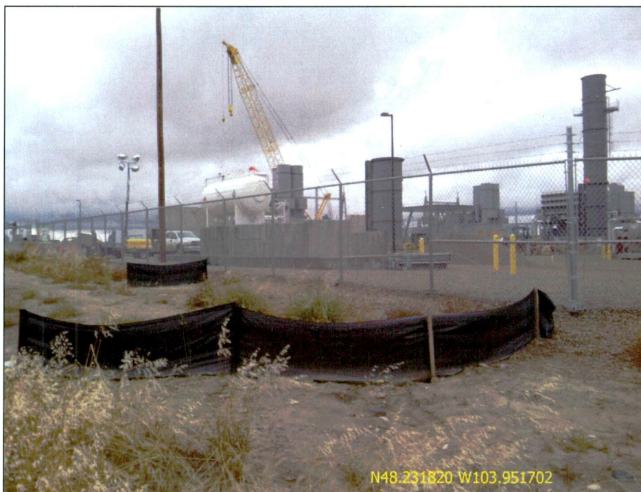
Figure 1. Photo taken looking northwest from the east side of the fenced area of the Pioneer Generation Station. Silt fencing was installed and working effectively.
