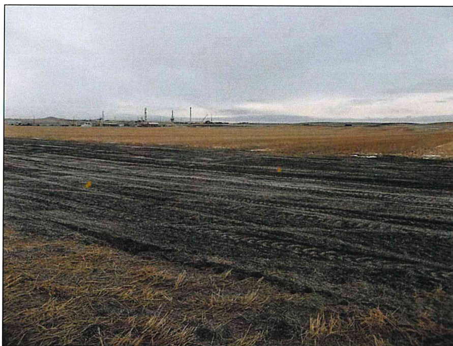
Figure 3. Project area overview depicting general topography, facing southwest, showing existing Garden Creek Gas Plant in background.
