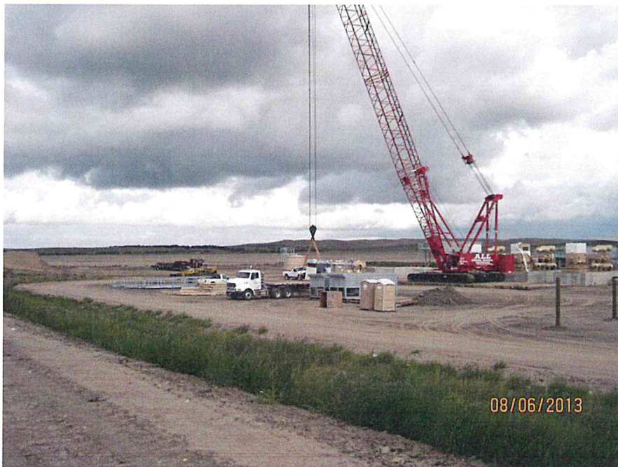
Figure 3. View from the western edge of Garden Creek II looking northeast
