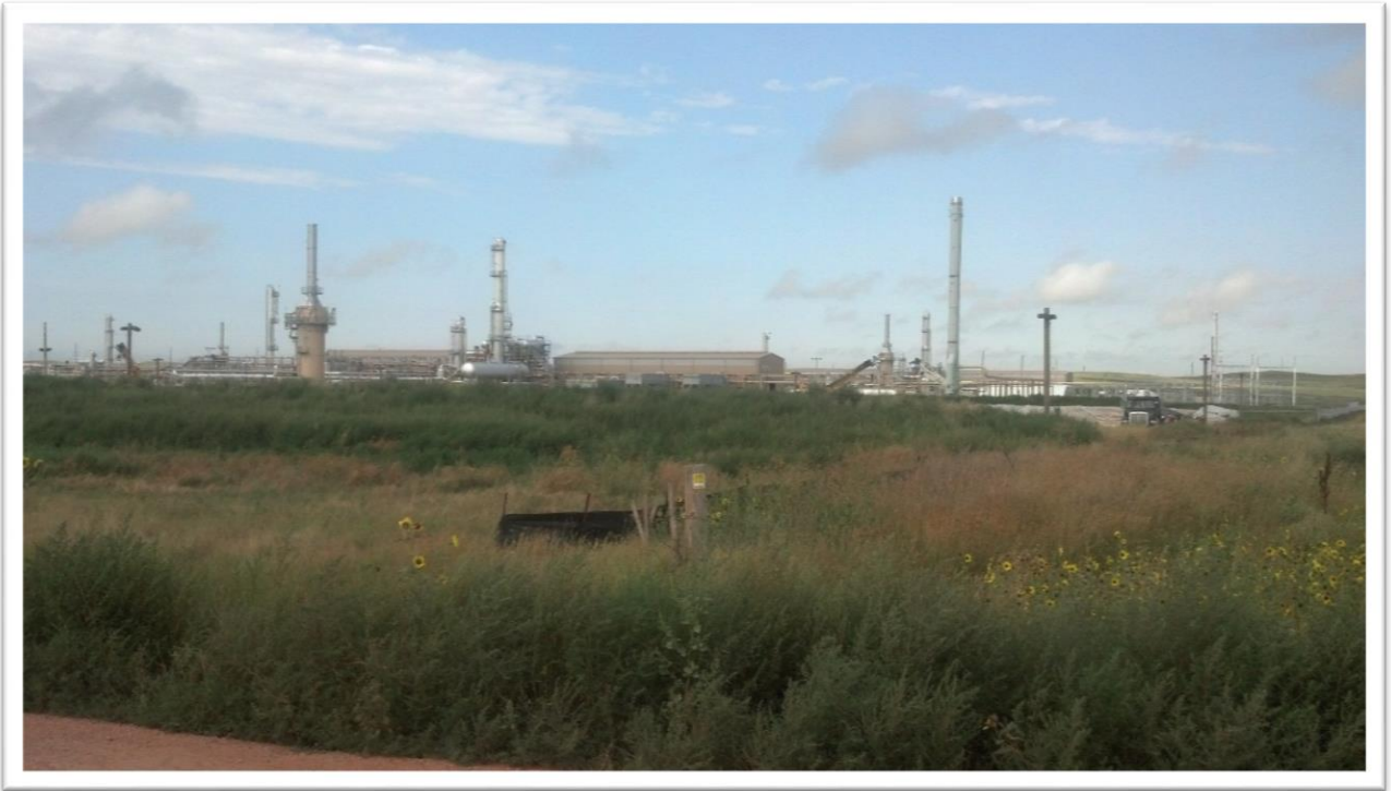
Figure 1. View from the northeast corner of GC III looking southwest
