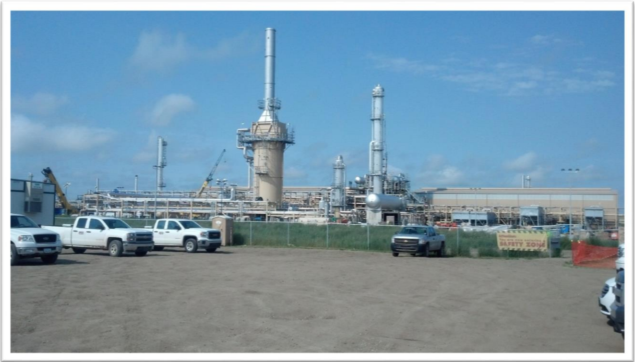
Figure 5. View near the east border of Garden Creek III looking west
