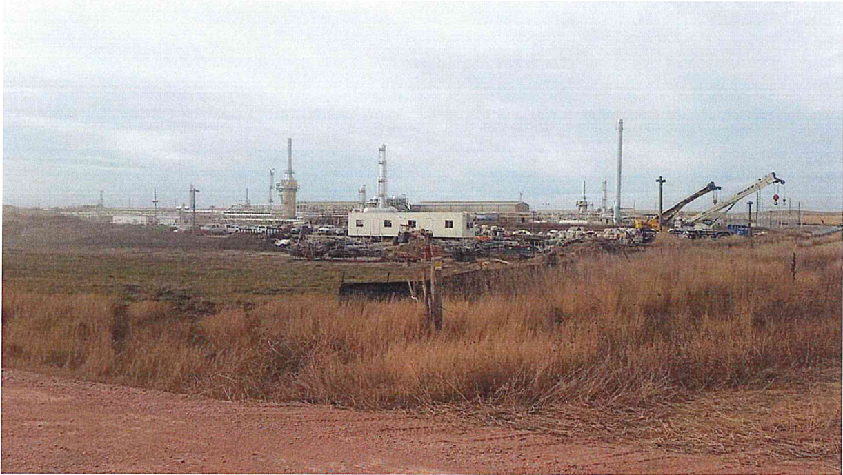
Figure 3. View of GC III near the northeast corner of GC III looking southwest
