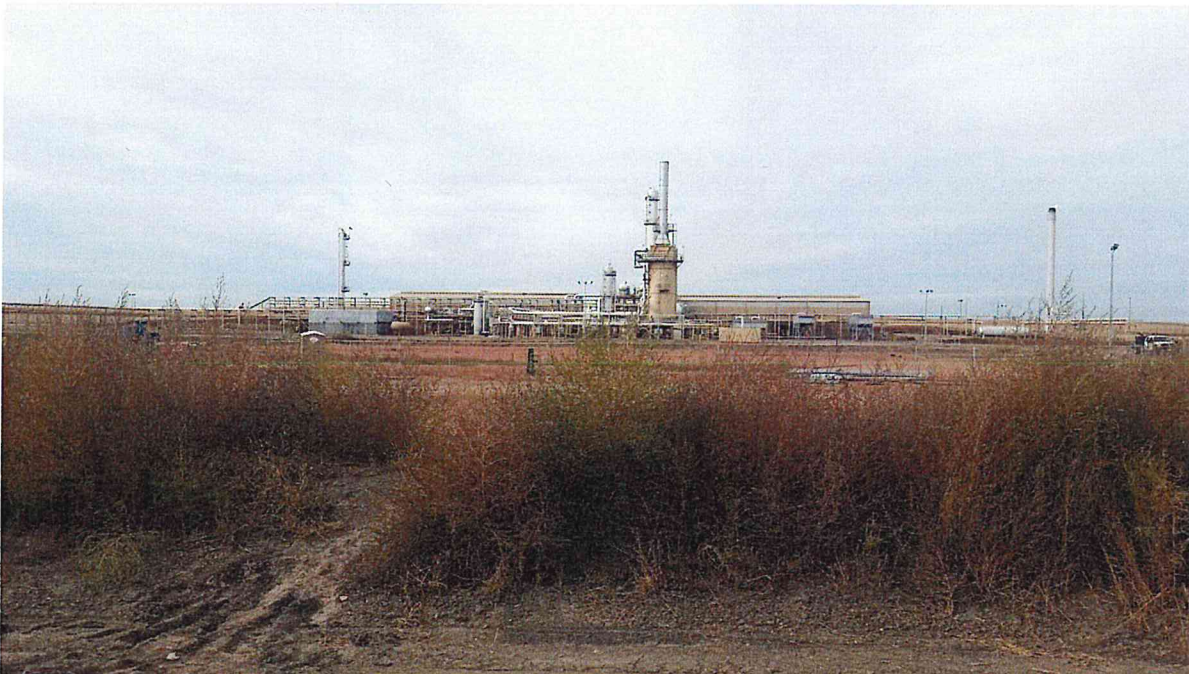
Figure 2. View from the east boundary of GC III looking west
