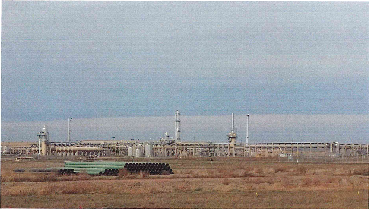
Figure 1. View from the southeast corner of GC III looking northwest
