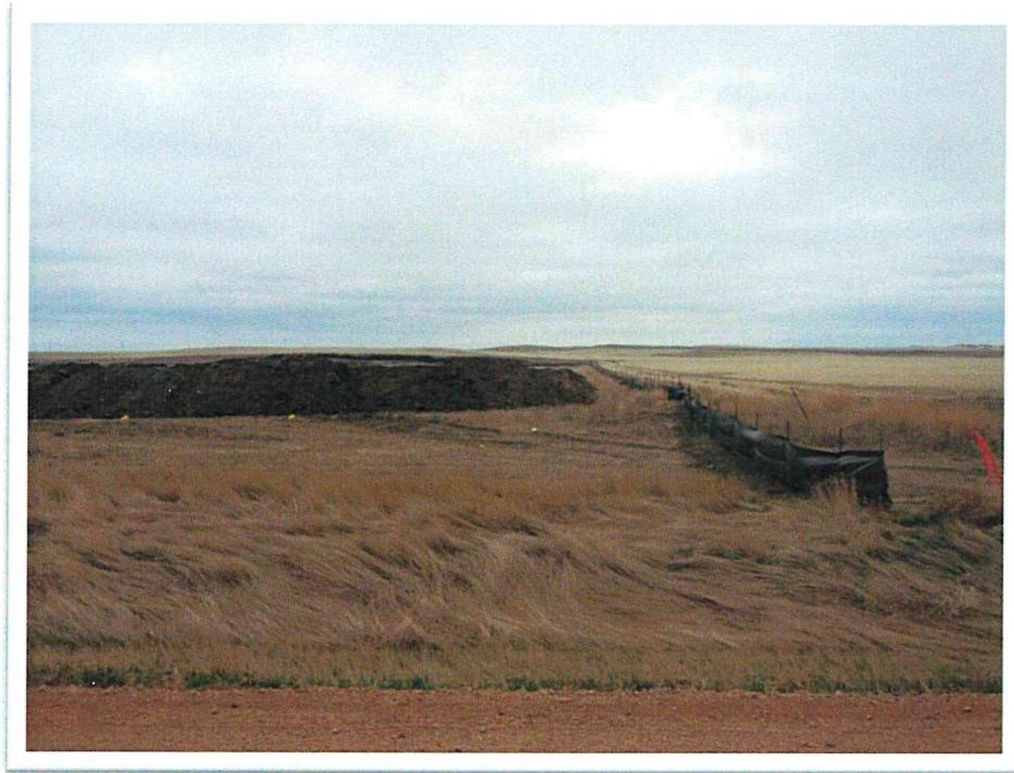
Figure 4. View from northeast looking west. Silt fence installed along north property line.
