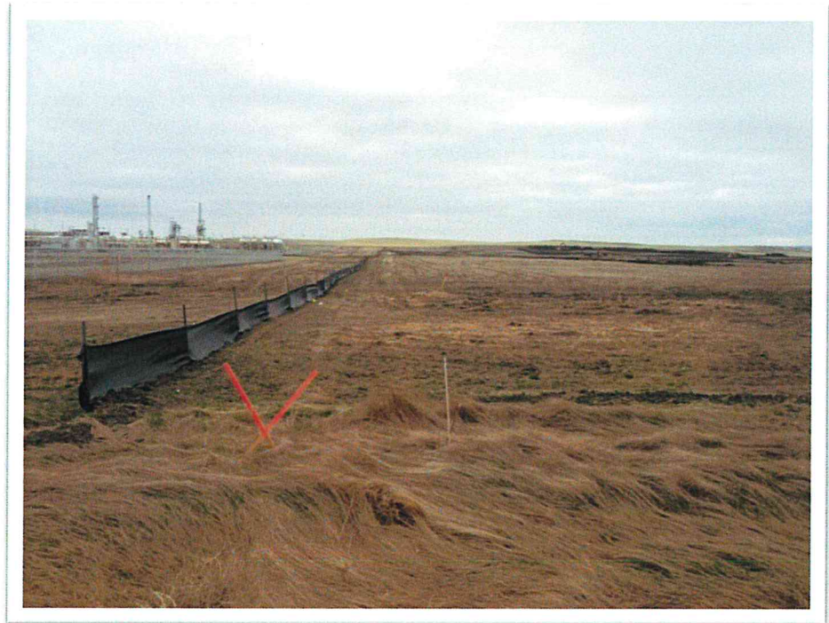
Figure 4. View from northeast looking west. Silt fence installed along north property line.
