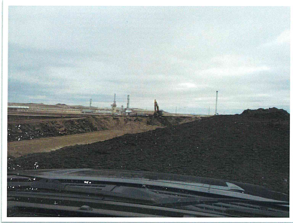
Figure 8. View from the northwest looking south at the site grading efforts.
