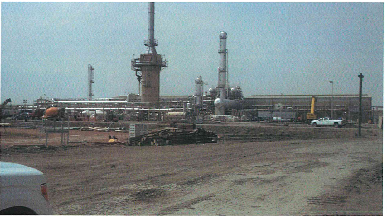
04/22/2014 Photo 20. View of GC II from the dividing line looking west.
