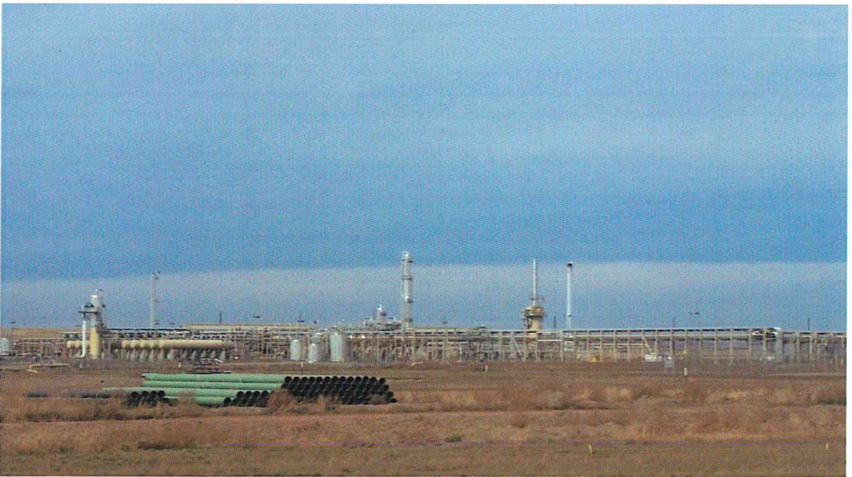
10/15/2014 Photo 26. View from the southeast corner of GC III looking northwest.
