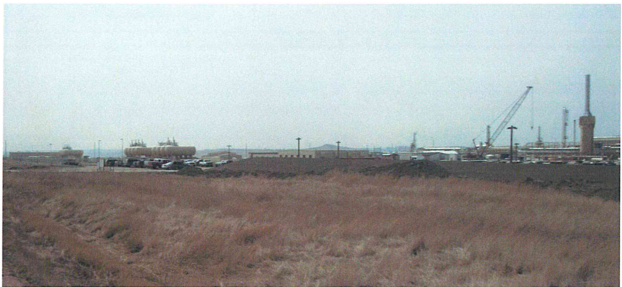
04/22/2014 Photo 14. View from the northeast corner of GC III looking southeast.
