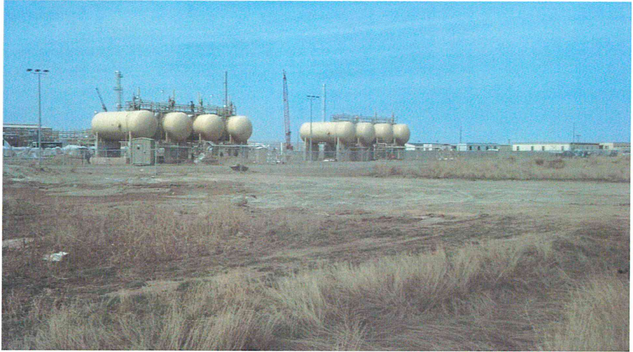
04/22/2014 Photo 17. View from the southeast corner of GC II looking northwest.
