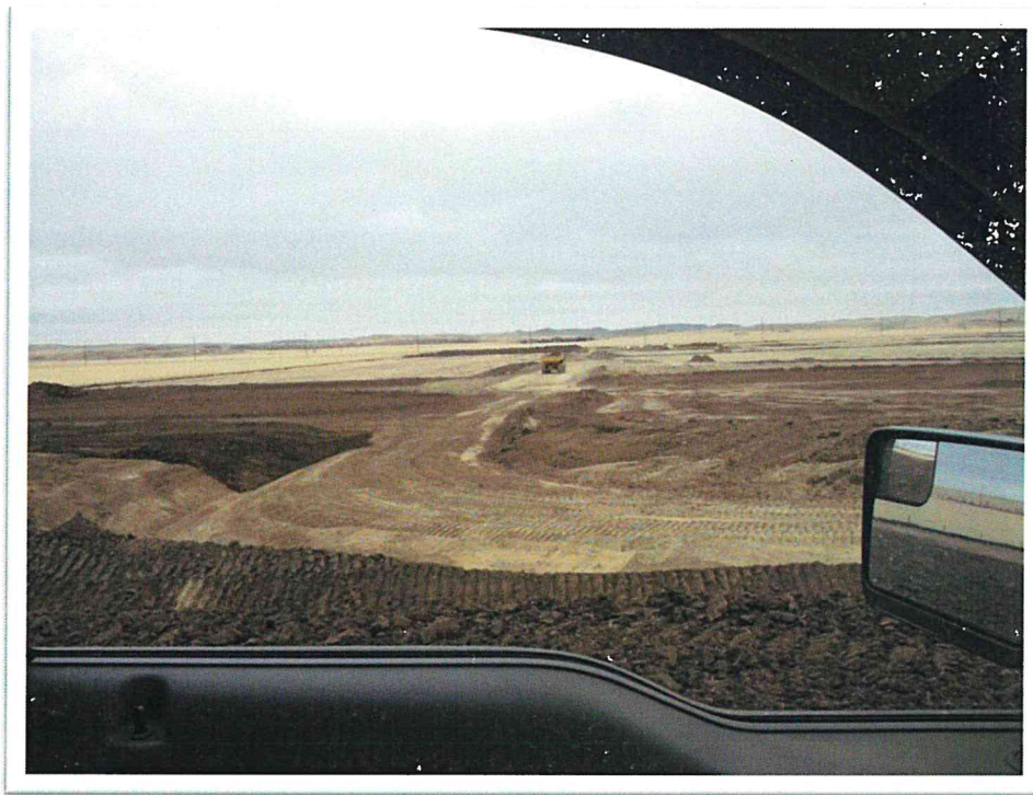
Figure 6. View from west looking east. Site roadways established. Silt fence along southern boundary is seen in the photo.
