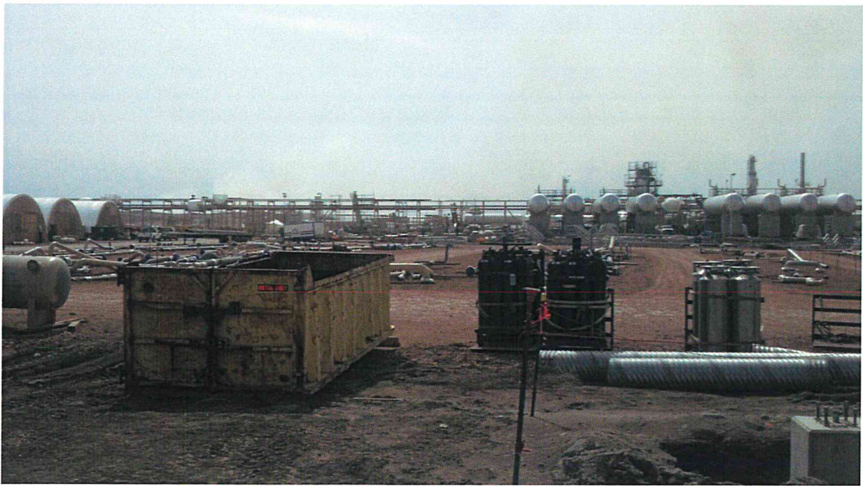
04/22/2014 Photo 18. View looking south at the dividing point between GC II & III.
