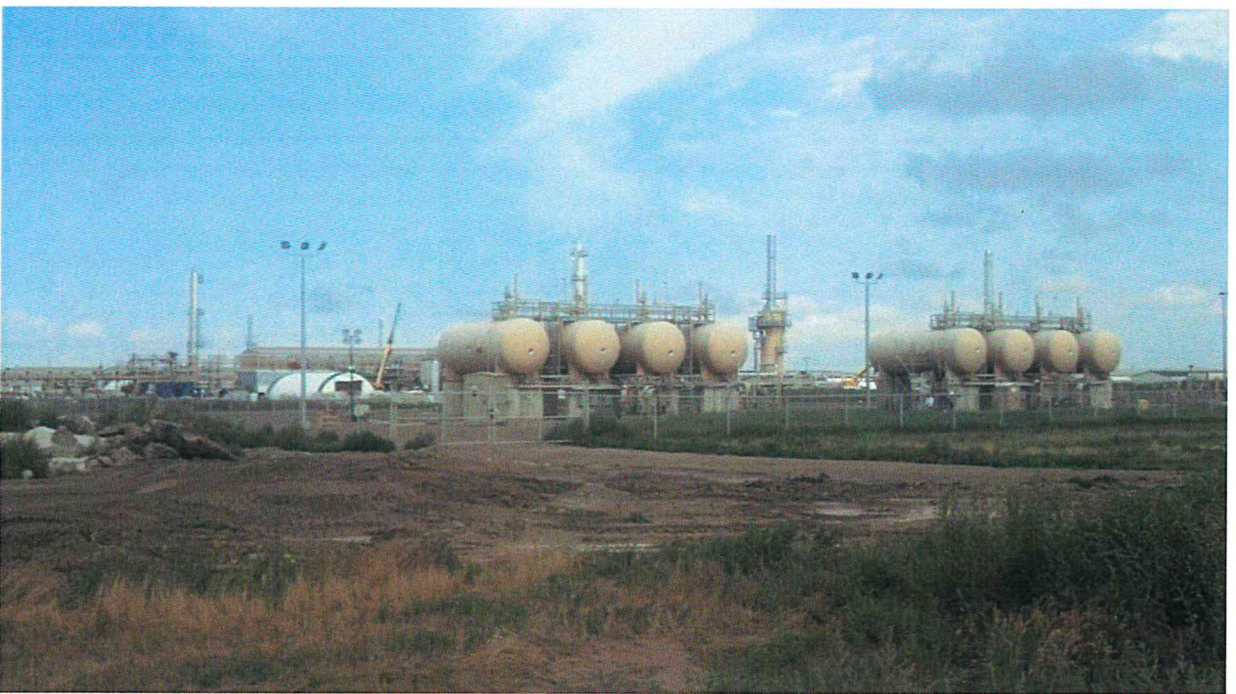
08/04/2014 Photo 22. View from the southeast corner of GC III looking northwest.
