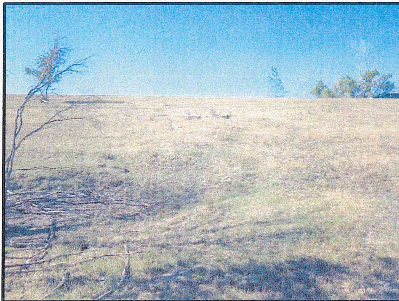
Photo 4. Direction: Northwest. View of the west end of Wetland 2. Note that there is no culvert under the road embankment.
