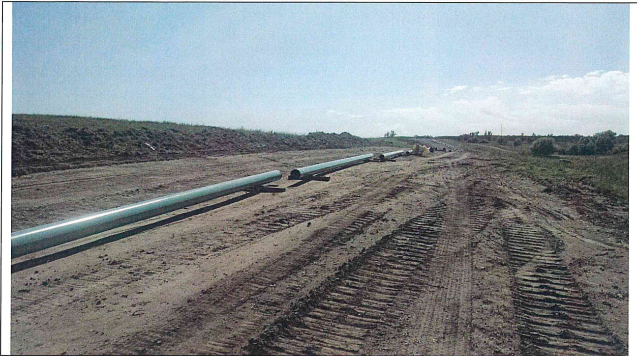
Photo 1: Pipeline laid out, Pipeline laid out, ready for permanent placement.
