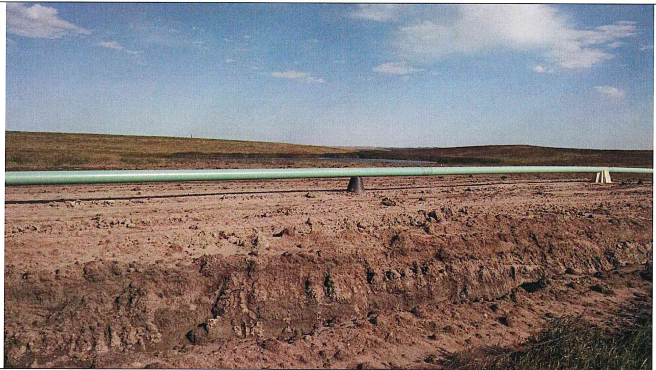
Photo 6: Pipeline laid out, ready for permanent placement.
