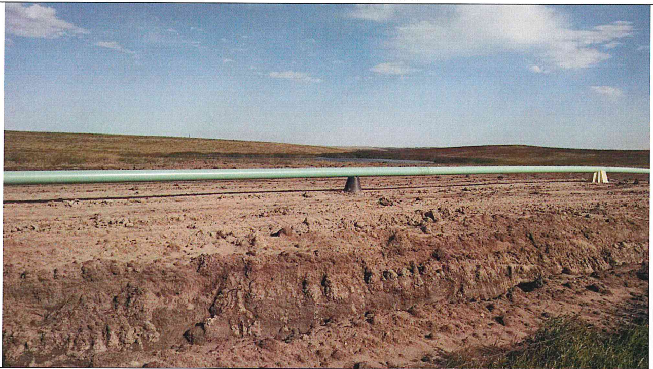
Photo 6: Pipeline laid out, ready for permanent placement.
