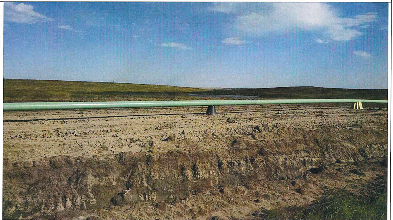
Photo 6: Pipeline laid out, ready for permanent placement.
