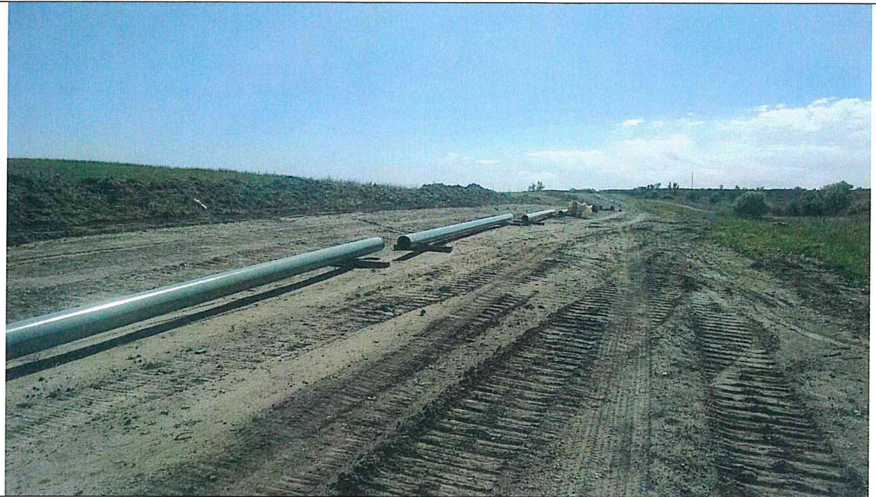
Photo 1: Pipeline laid out, Pipeline laid out, ready for permanent placement.
