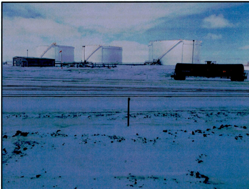
Photo 6. Direction: North. Another view of pipeline ROW toward rail terminal pig launcher on north end of Project. An additional pipeline ventilation marker is visible in foreground.
