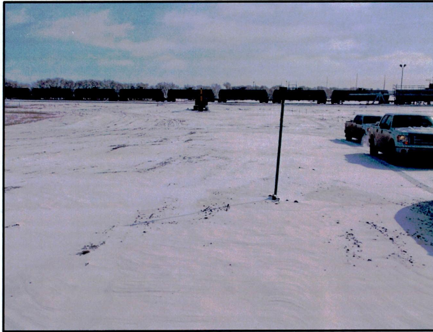
Photo 5. Direction: North. Pipeline ROW north toward rail terminal pig launcher on north end of Project. One pipeline ventilation marker is visible in foreground.
