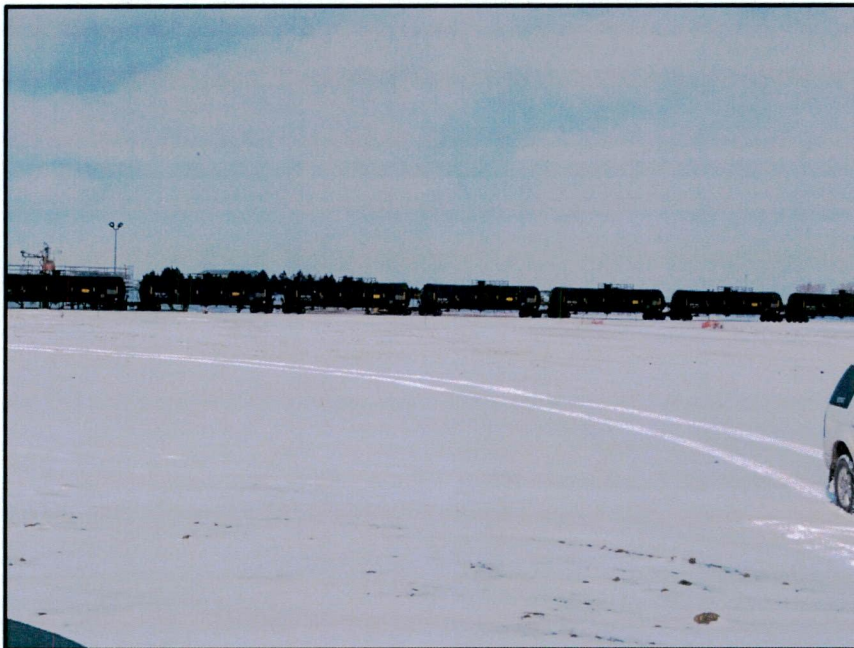
Photo 4. Direction: North. Pipeline running toward Tioga Rail Terminal on the north end of the Project. Additional view of area that still needs to be reclaimed.
