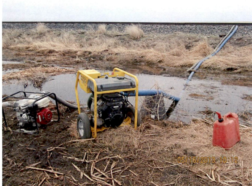
Photo: 5: Use of pumps and gas can within mapped wetland; no secondary containment or spill measures in place. Taken to the east of 89 th Ave. NW where pumping activities were occurring at time of inspection.
