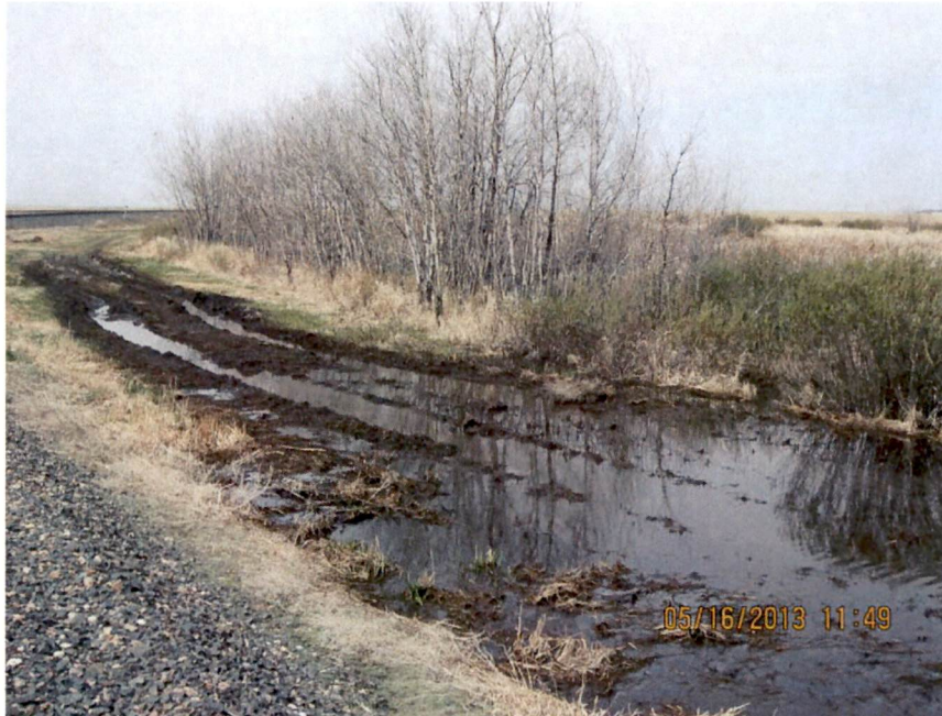
Photo: 3: No erosion or sediment control devices in place to protect wetland in the background.
