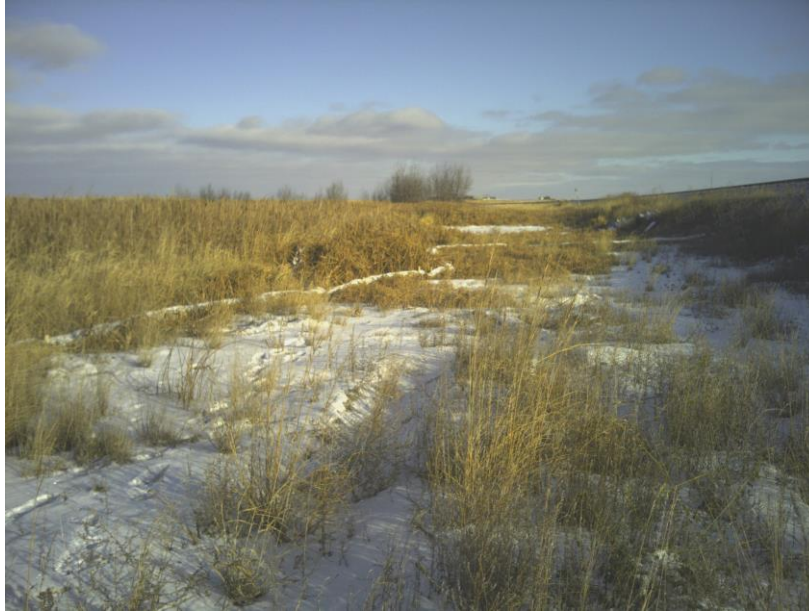
Photo 4: Straw wattle still present at STA 40+00, straw wattles may be left in place provided they degrade naturally over time
