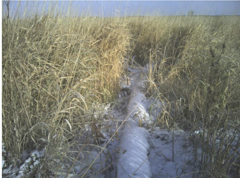
Photo 1: Straw wattle still present at STA 347+85 and 352+49, straw wattles may be left in place provided they degrade naturally over time.
