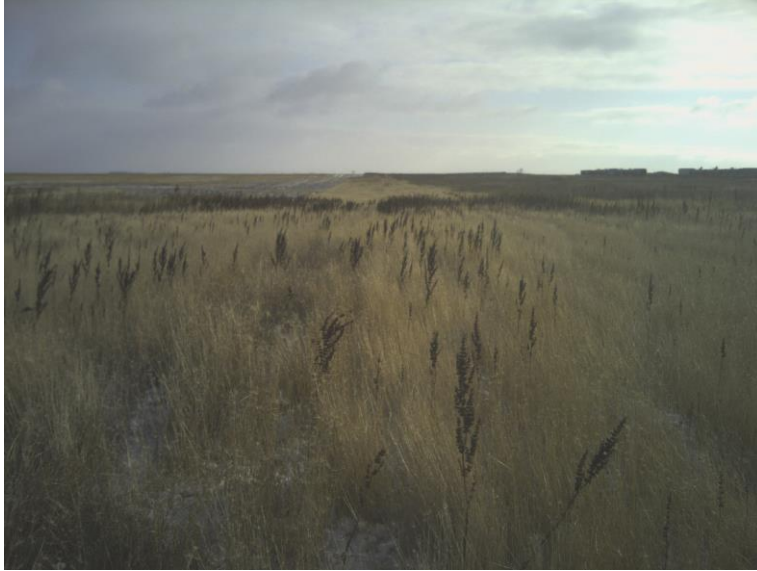
Photo 2: Looking east along pipeline right-of-way near STA 340+00. Final stabilization has been achieved.
