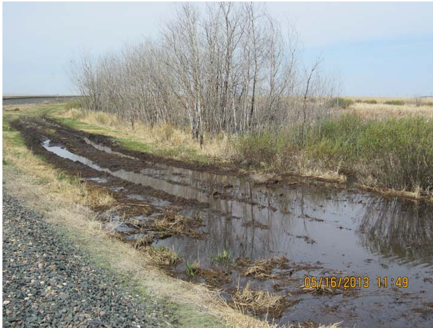
Photo: 3: No erosion or sediment control devices in place to protect wetland in the background.
