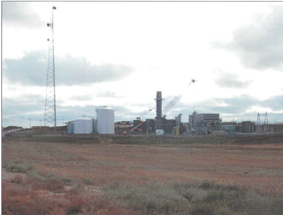
Figure 1. Overview of BEPC Lonesome Creek Station. Phase I turbine is operating while Phase II construction is in progress.
