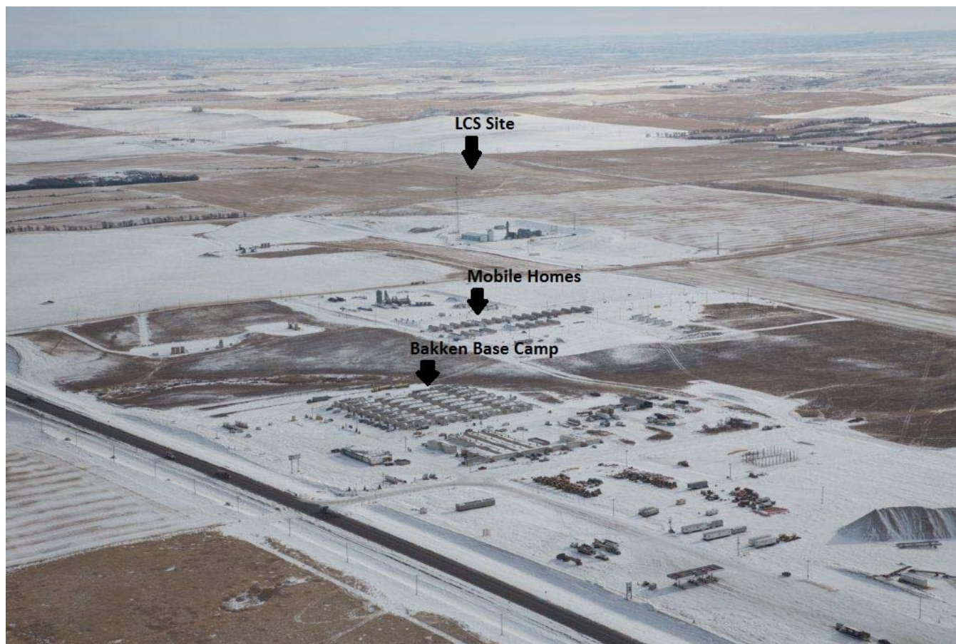
Figure 2-2: Aerial view of the Bakken Base Camp and Mobile Homes in Comparison to LCS
