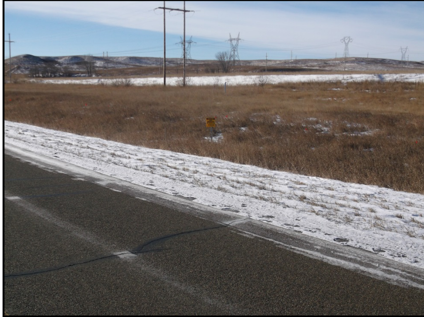
Photo 15. Direction: Northeast. This is the entry point for the third bore of the project underneath County Road 15. An above ground pipeline yellow marker shows the entrance point of the bore. During the inspection no impacts to the road were observed.
