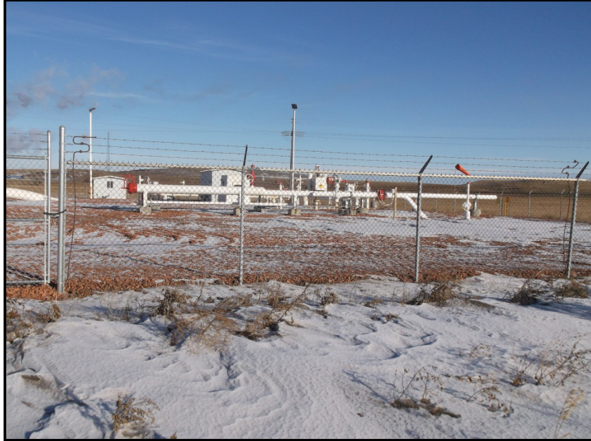
Photo 1. Direction: East. Pig launcher located on the south end of the project. The pipeline then proceeds west underneath County Road 26. Some reseeding is still required; it is expected to be completed this spring. This was the only area within the project limits where vegetation had not been established.
