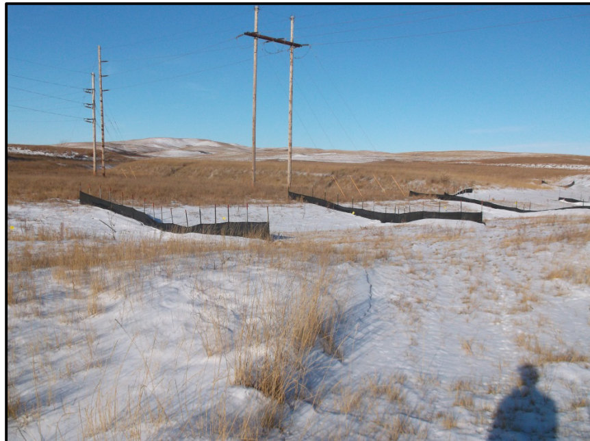
Photo 12. Direction: Northwest. BMP's are still in place along pipeline corridor to prevent against erosion during this downhill portion of the corridor, where a channel has been created.
