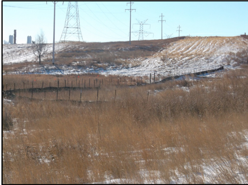
Photo 11. Direction: South. Silt fence encompassing one of the wetlands along the pipeline corridor. The silt fence has remained installed to continue to protect the wetland. During the inspection no impacts to the wetland were observed.
