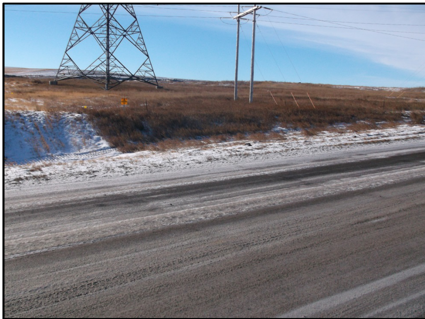
Photo 6. Direction: South. 4 th St SW (County Road 26) bore. Yellow marker indicates location of the start of the bore. No impacts to the road were observed during the inspection.
