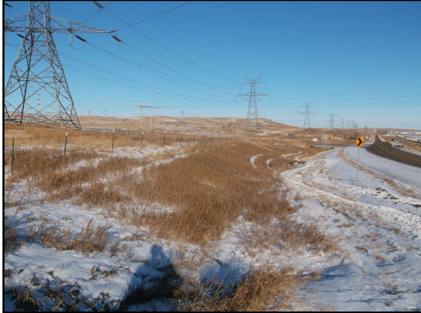
Photo 5. Direction: North. Pipeline is still bending towards north bound route in this photo and it is approaching the second boring of the job underneath 4 th St SW (County Road 26).
