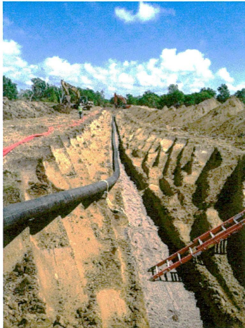
8-05 Low quality water pipeline
