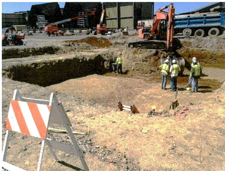
8-09 Excavating ID fan area
