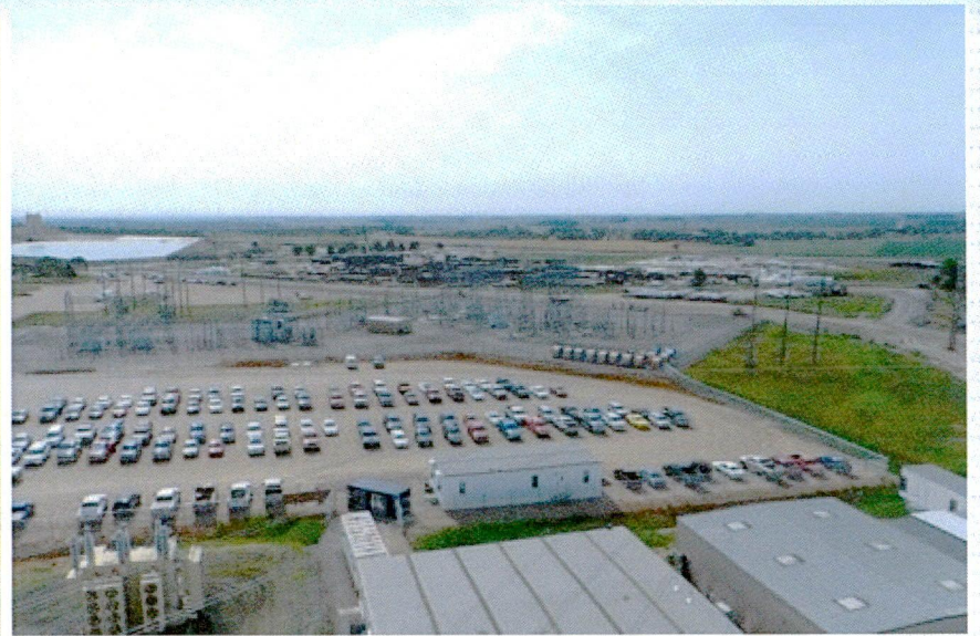
8-21 Main laydown area, contractor parking lot, office complex
