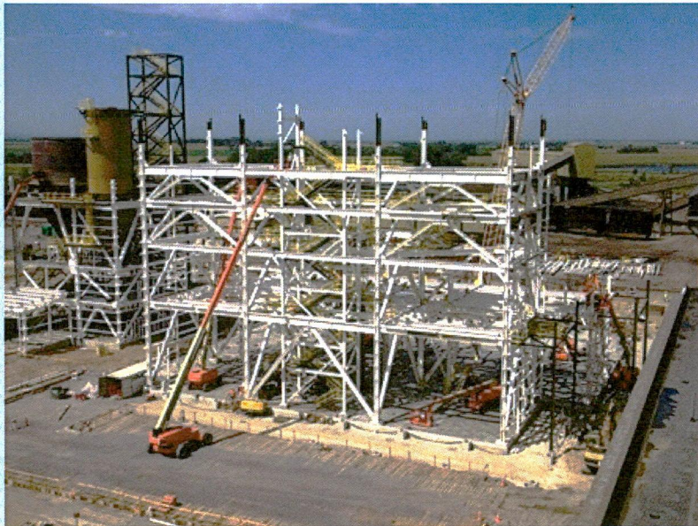
8-29 CFB & start of baghouse steel erection
