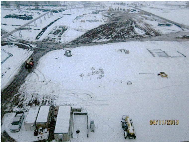
4-11 South view - working in early spring snow!
