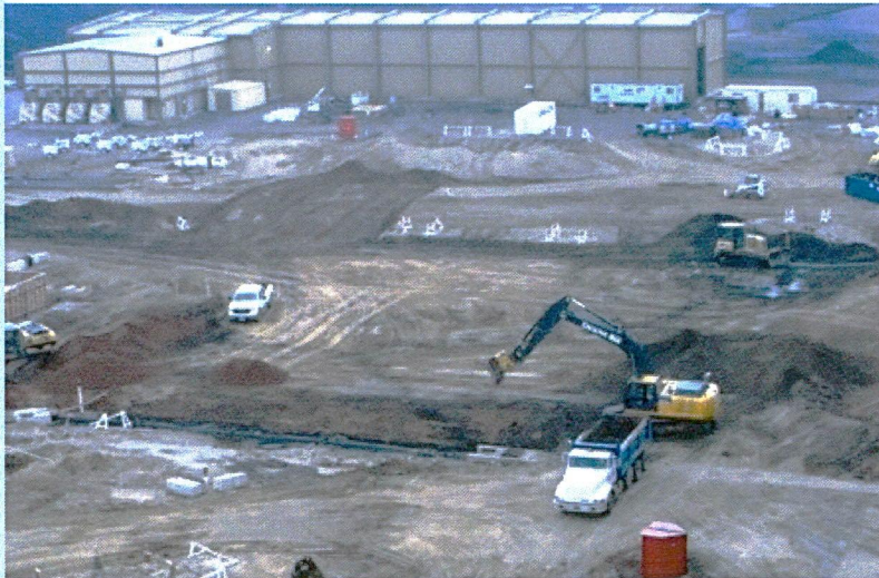
5-29 Baghouse and CFB excavation
