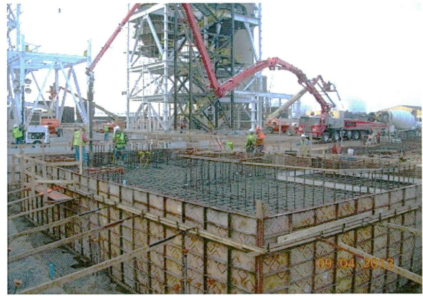
ID Fan B foundation placing concrete
