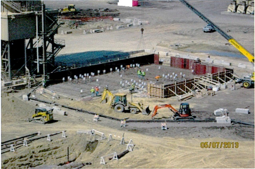
5-07 Foundation rebar placement
