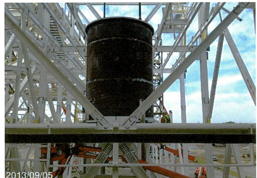
9-05 Waste ash bin lowered
