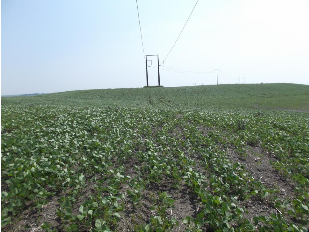
Above: Photo 19 (Observation Point 18) – Near connection to existing structure at northwest corner of project. Looking east.
