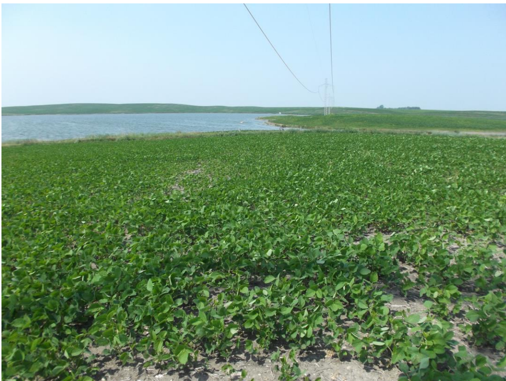
Below: Photo 20 – Existing transmission line at northwest corner of project. Looking west.
