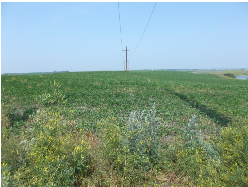
Below: Photo 16 (Structure 0685B) – Typical vegetation between new structures. Looking northwest.
