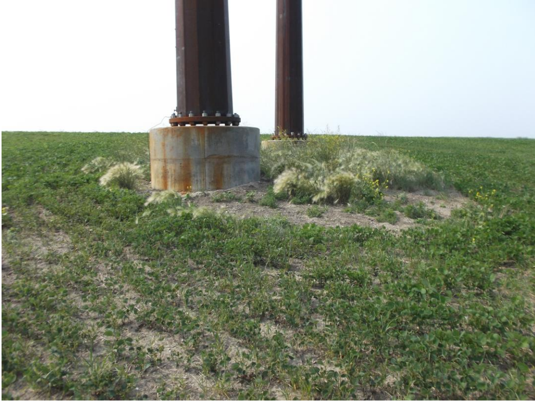
Above: Photo 7 – Typical vegetation around structure. Grass and weeds within 5 to 10 feet of base, but crop growing in surrounding area. Looking south.
