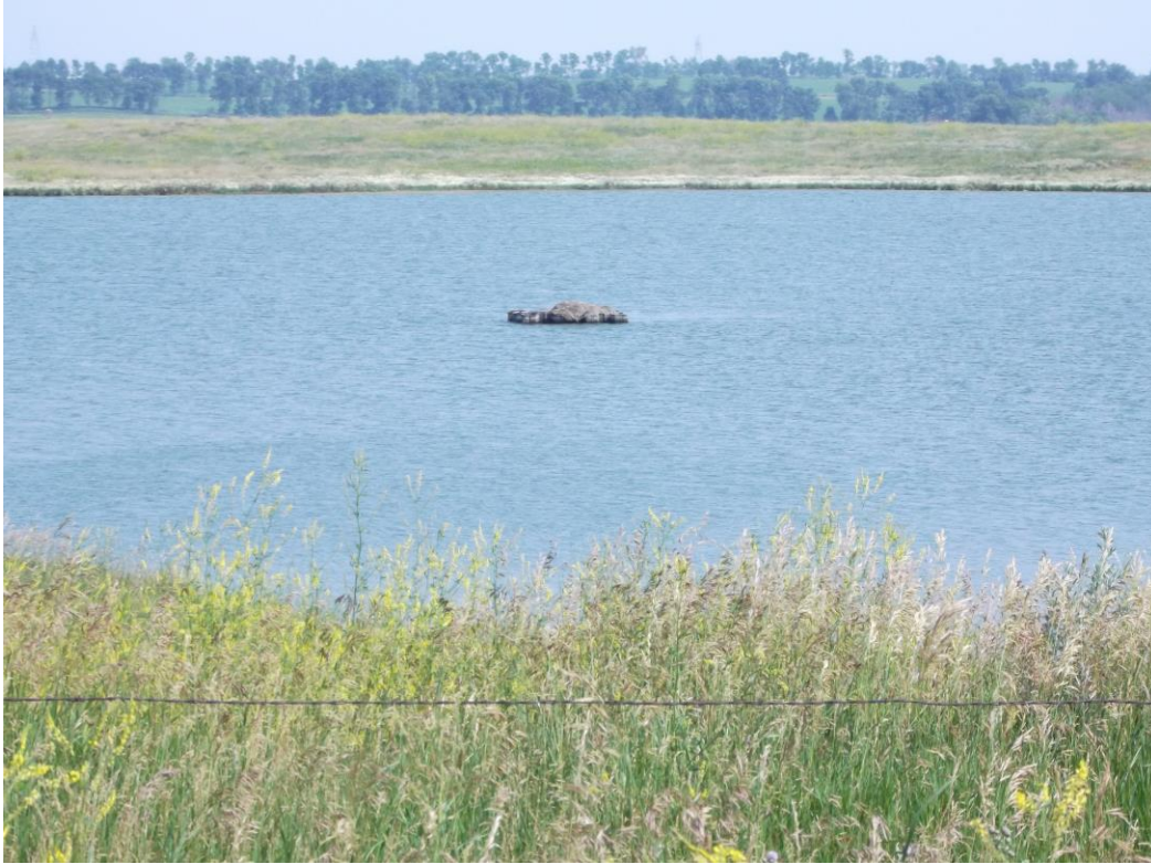
Above: Photo 15 (Observation Point 14) – Apparent abandoned/removed structure in wetland. Looking north.
