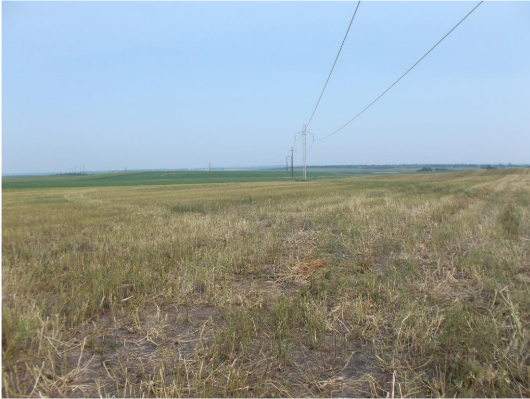
Above: Photo 1 (Observation Point 1) - Connection to existing transmission line structure at south end of Project. Looking northwest.
