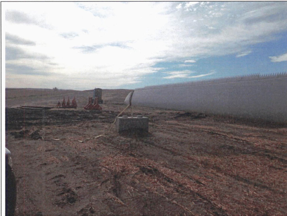
Photo 3: Site 457, showing turbine laydown area.
