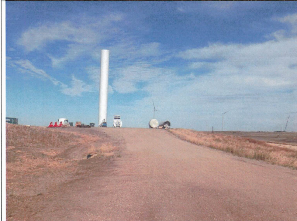
Photo 4: Site 433, actively under construction.
