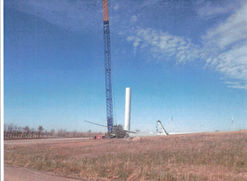
Photo 6: Active construction on pad for turbine 452.
