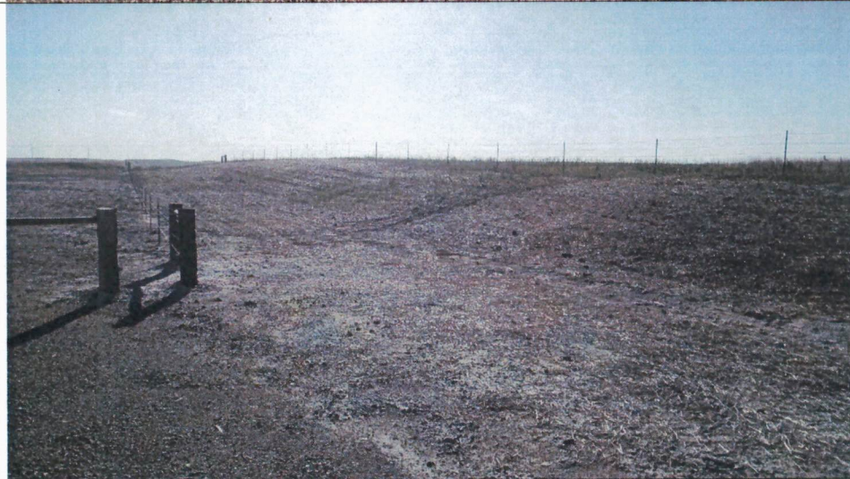
Photo 3: Partial revegetation of area near Turbine 441
