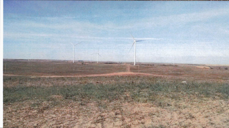
Photo 6: revegetated collector line ROW.
