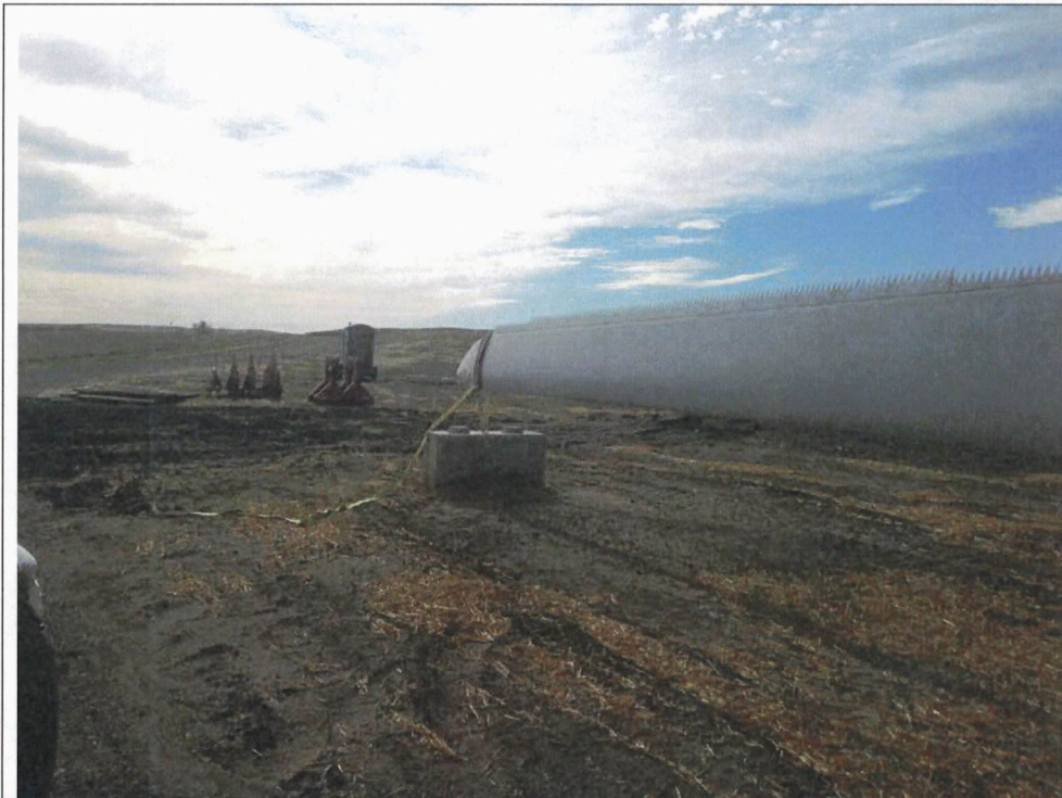
Photo 3: Site 457, showing turbine laydown area.
