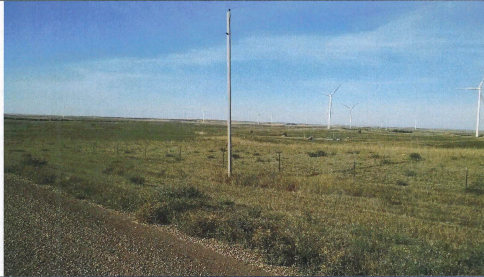
Photo 1: Looking west from 57 th Ave at Collector line crossing. Turbine 451 is on the right of the photo.
