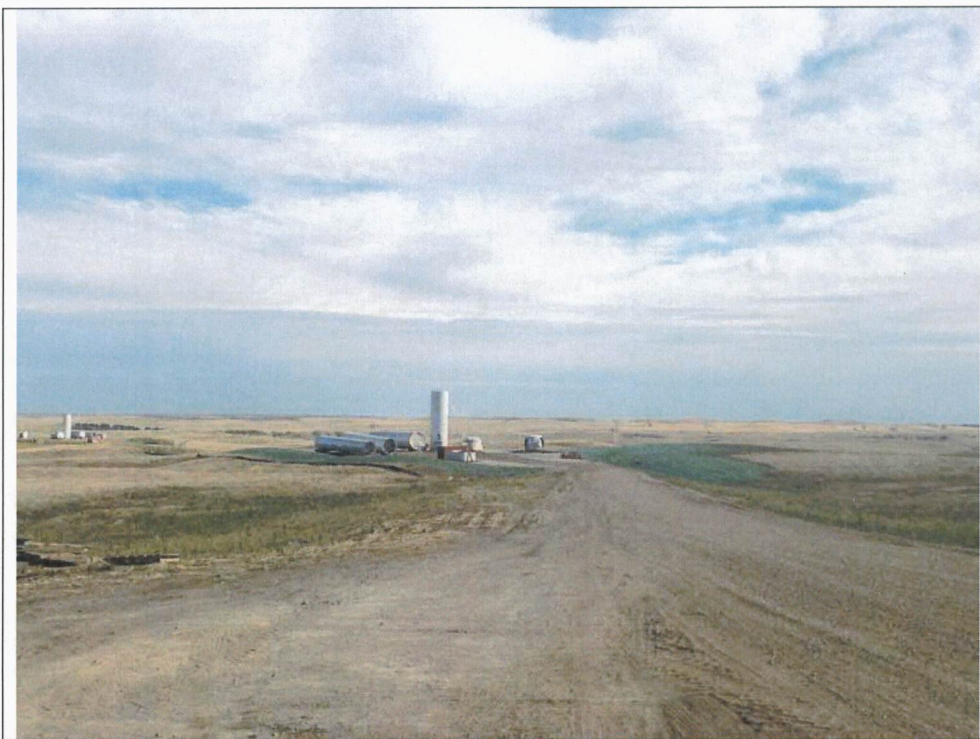
Photo 7: Site 439, recent hydroseeding.
