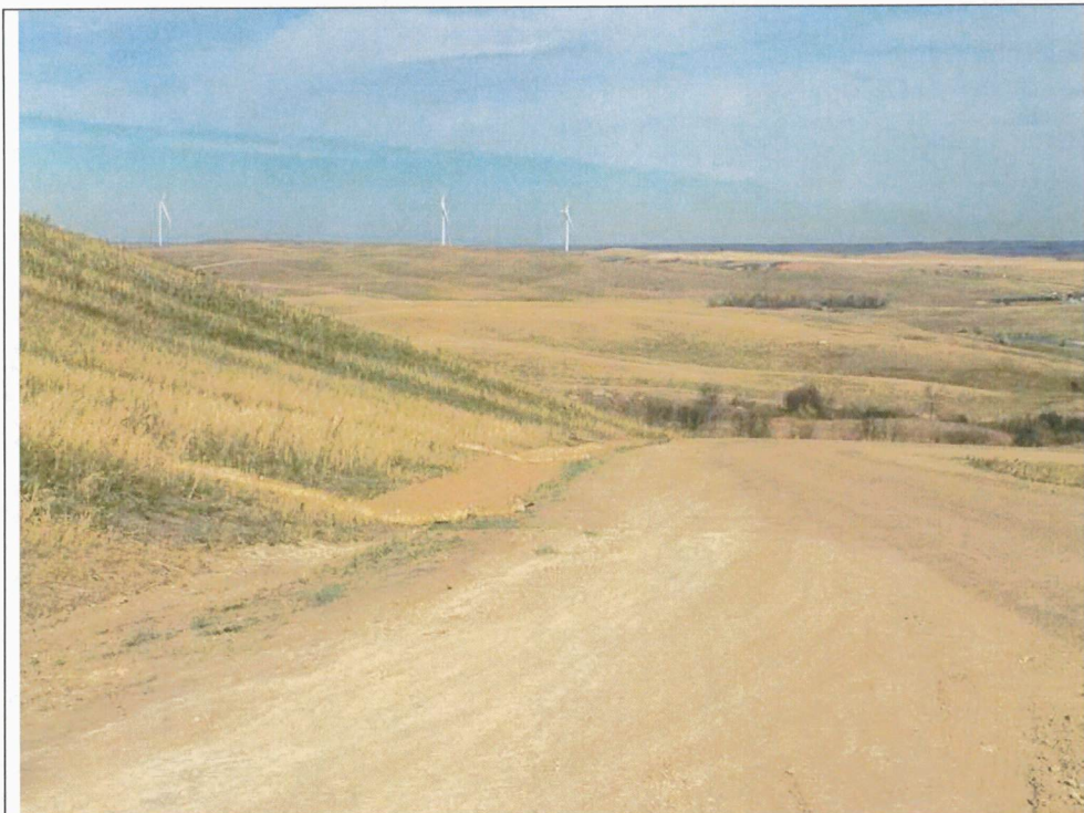
Photo 1: Site 421, showing erosion control measures.
