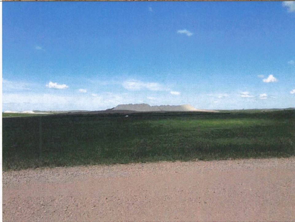
Photo 6: Active construction on pad for turbine 420. Silt fencing observed surrounding pad.
