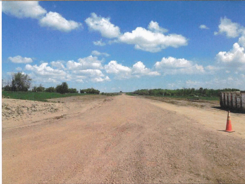
Photo 8: Completed access road for turbine 421, from the south facing north.
