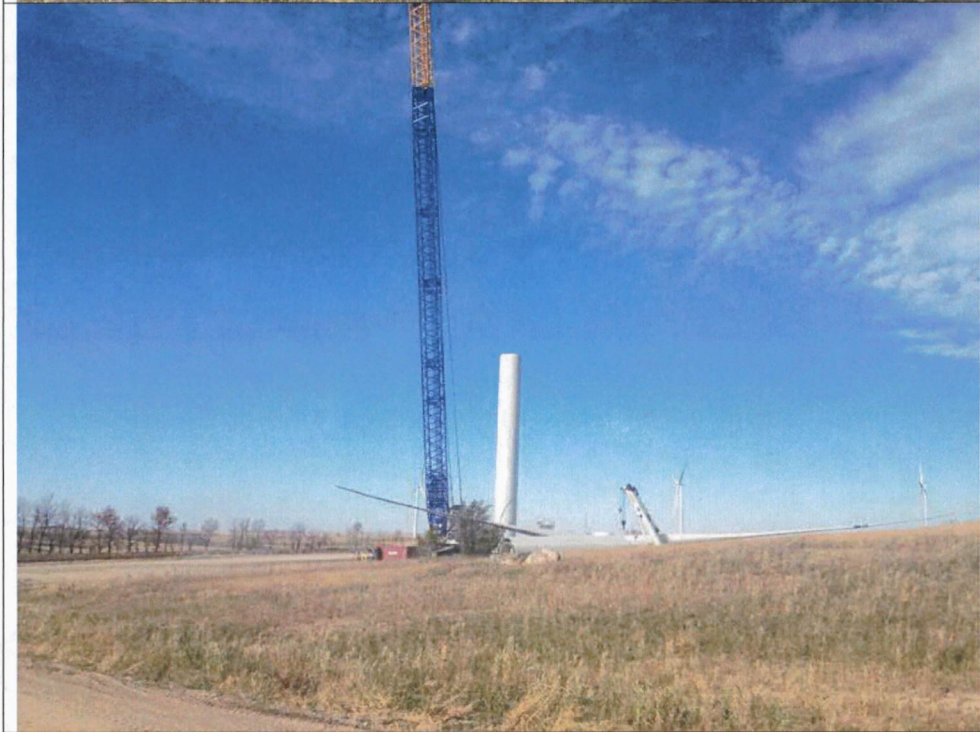
Photo 6: Active construction on pad for turbine 452.
