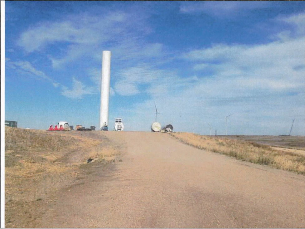
Photo 4: Site 433, actively under construction.
