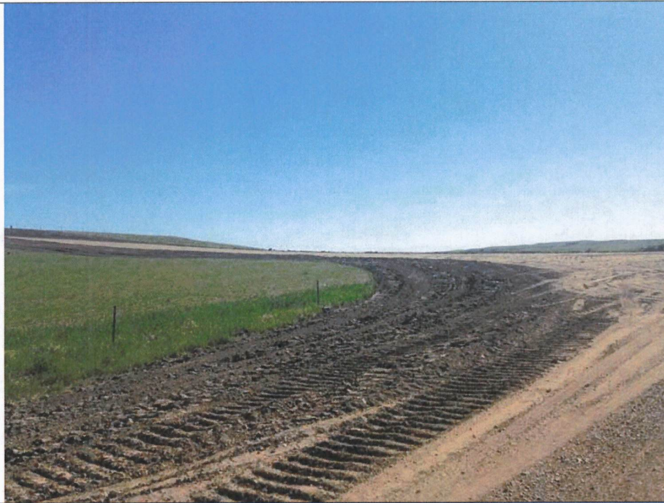
Photo 3: Access road for turbine 462. The county road conditions in this area were relatively rough, however active construction equipment was in the area. This roadway will need to be restored to the original condition.
