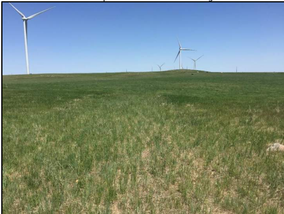
Photo 7. Facing: Northeast. Location: 47.018928, -101.706300 View along the collector line southeast of T449. T451 is visible in the northwest corner of the photo. This area had the least vegetation cover observed along the route, but still had a satisfactory stand of seeded native grasses that will continue to establish over time without intervention.
