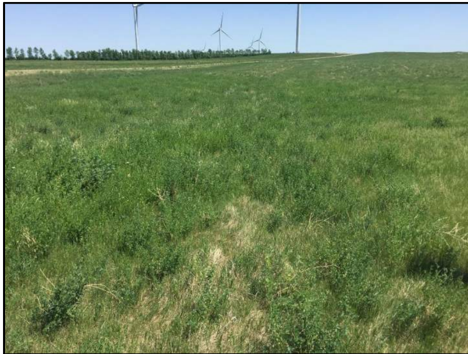
Photo 2. Facing: Northeast. Location: 47.016456, -101.719680 View of the collector line between T448 and T449. The collector line scar is nearly indistinguishable compared to the surrounding landscape.
