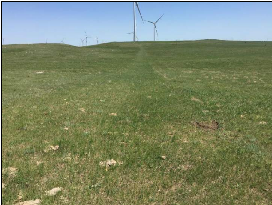
Photo 9. Facing: Northeast. Location: 47.021992, -101.710267 Overview of the collector line between T450 and T451 from the southwest end. The route of this line is nearly indistinguishable to the surrounding area.
