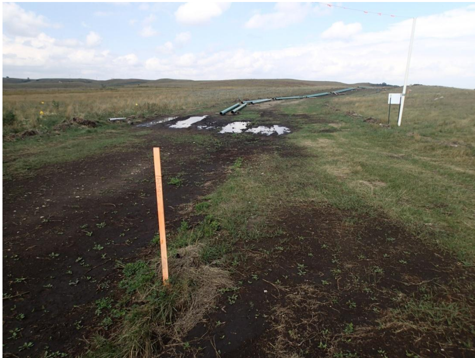
Figure 14. Pipeline. View to the north.
