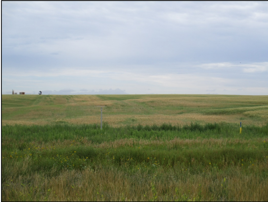
Photo 3. (GPS Point #13) Pipeline ROW through field. Pipeline marker/sign is missing the placard, with only the metal pole standing (in center of photo). Yellow and blue pipeline marker to the right of photo. Good vegetative growth in crop field comparable to adjacent part of field. Direction: East.
