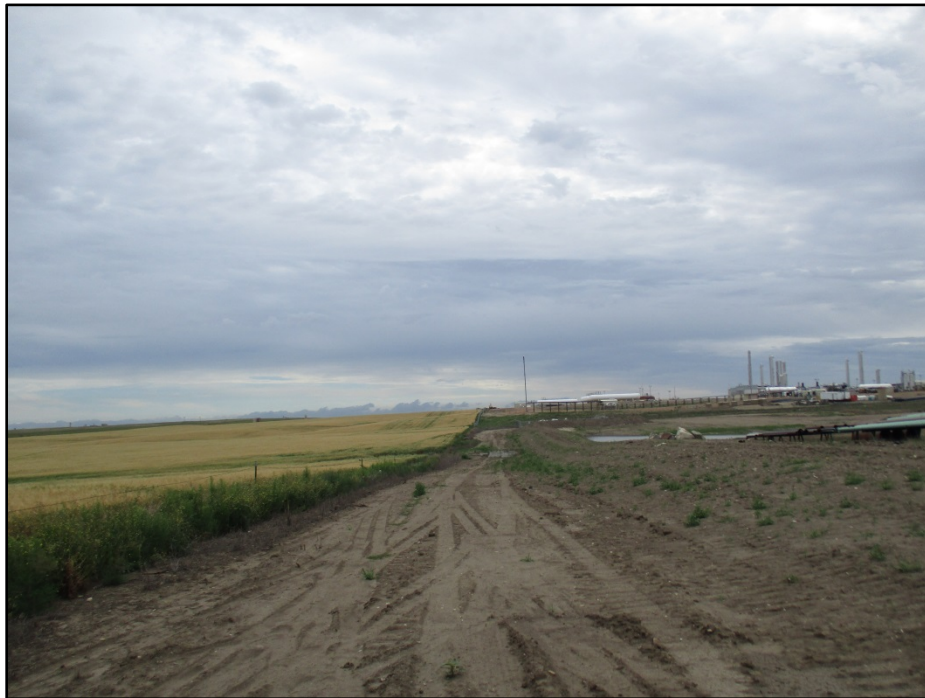
Photo 2. (GPS Point #10) – Dore Junction area. Berm (to the right of photo) was put up to stop stormwater runoff to the adjacent farmer's field.
