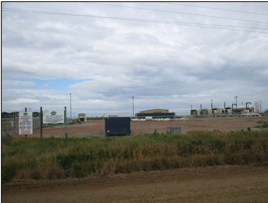
Photo 4. (GPS Point #14) – West Camp Creek Injection Station. Area is fenced and has signs. Direction: West.
