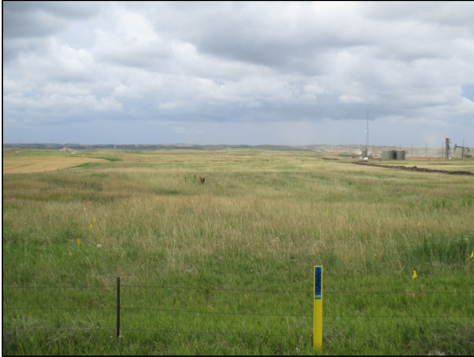
Photo 7. (GPS Point #17) – Area across from East Camp Creek Injection Station. Pipeline markers and flags in the ROW, flags due to nearby construction (seen to the right of photo). Direction: West.
