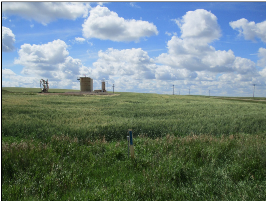
Photo 16. (GPS Point #36) – Pipeline ROW, goes through a crop field. Direction: South.
