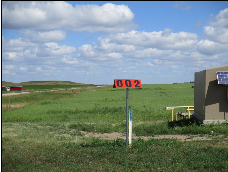
Photo 17. (GPS Point #36) – Pipeline ROW going though field. Direction: North.
