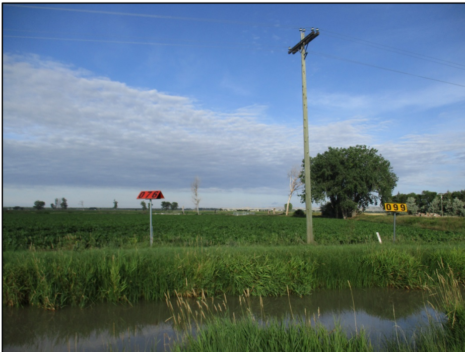
Photo 10. (GPS Point #23) – ROW bored under canal. Area is just west of river crossing. Valve station is fenced in the background. Direction: West.
