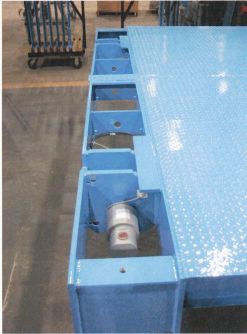
Cover Plates removed on both sides of one section.
