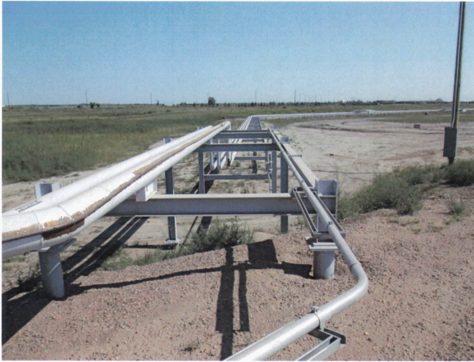
Above: Figure 5. Approach to bridge and river crossing on east side
