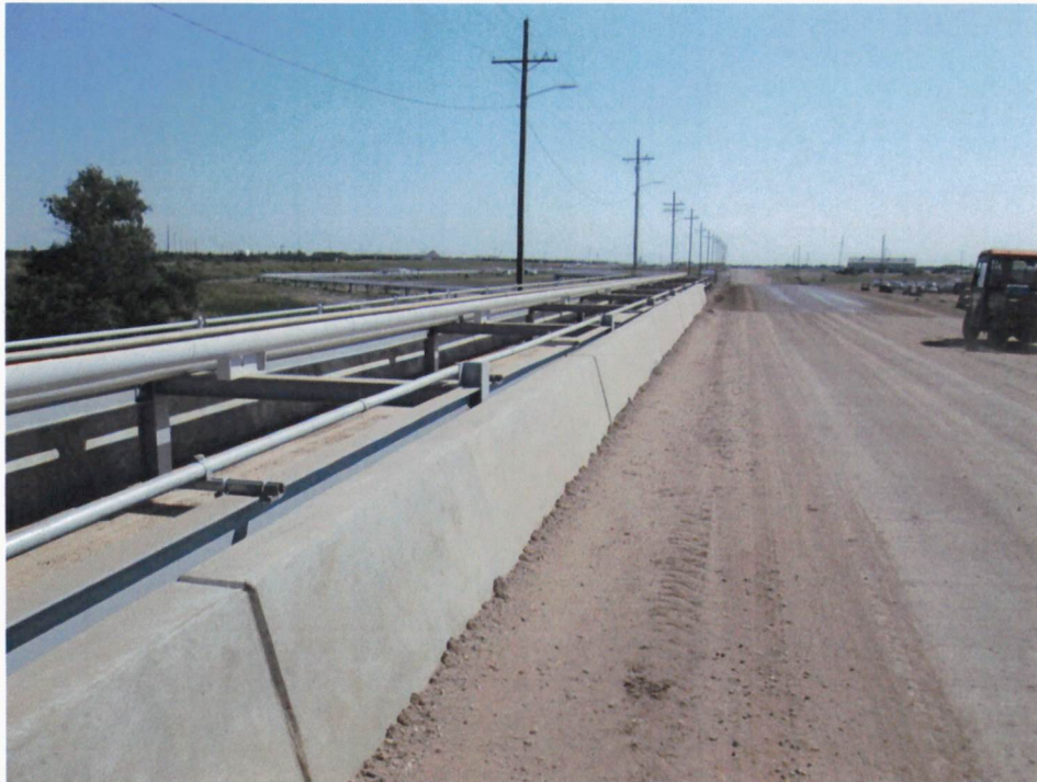
Below: Figure 6. Bridge Crossing Heart River
