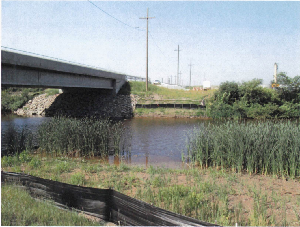
Above: Figure 7. Erosion control on the banks of the Heart River
