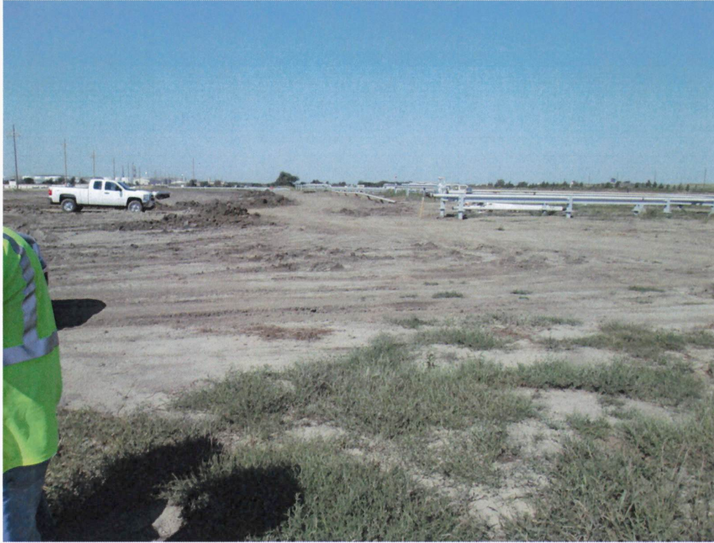
Above: Figure 3. Looking West along pipeline
