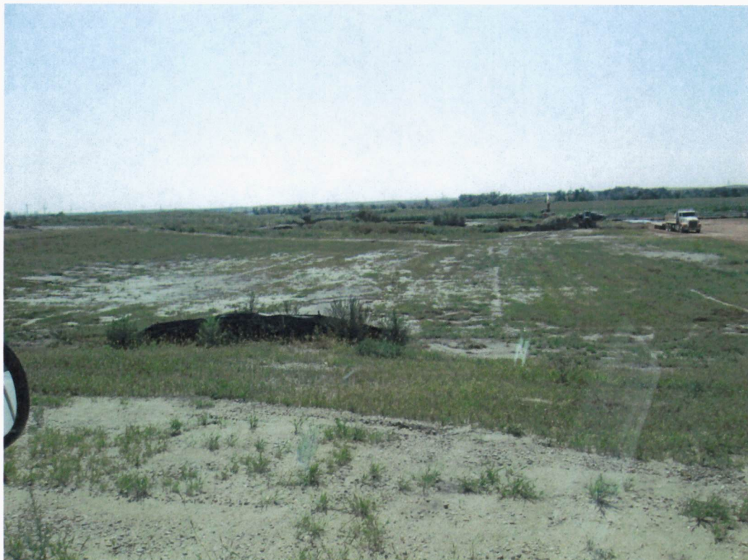
Below: Figure 8. South side of Entrance Road into Plant (Opposite Pipeline)
