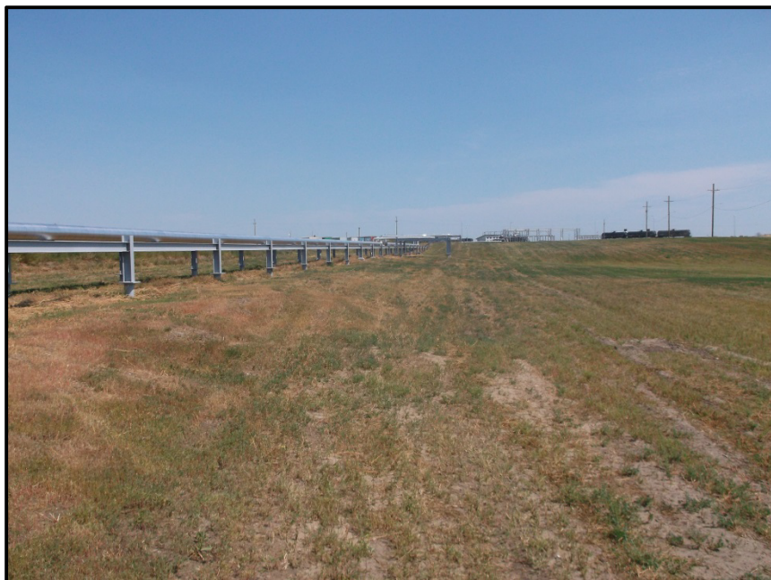
Photo 18. Direction: East. Depicted above is an example of the recovery of the ROW to preconstruction conditions. This section of pipe is north of the facility access road, runs east to west until it reaches the bore location at 116 th Ave SW. (This photo is from the second and final inspection of the pipeline).
