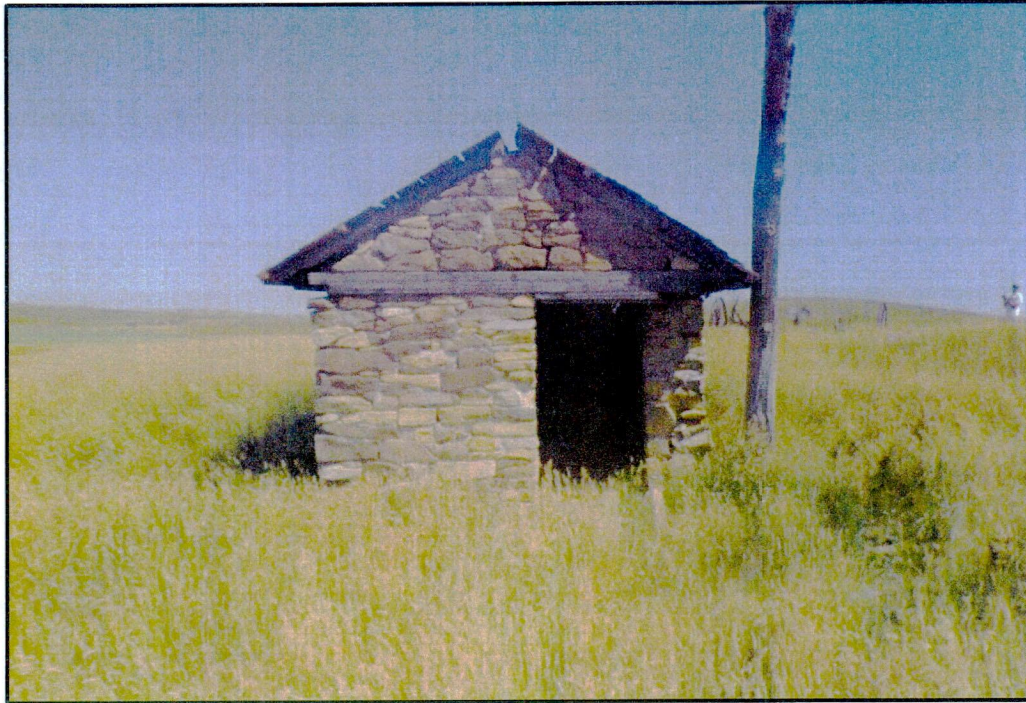
Figure 51: South end of smokehouse (Feature 1) from site 32SK1099, view north.
