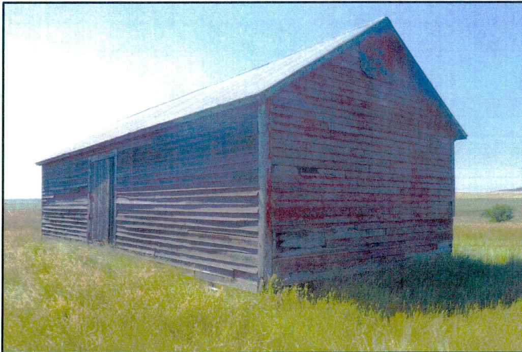
Figure 54: Northeast corner of Feature 2 from site 32SK1099, view southwest.
