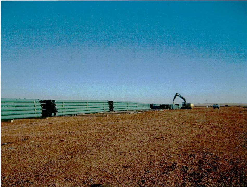
Photo 1 – Pipe Storage Yard
