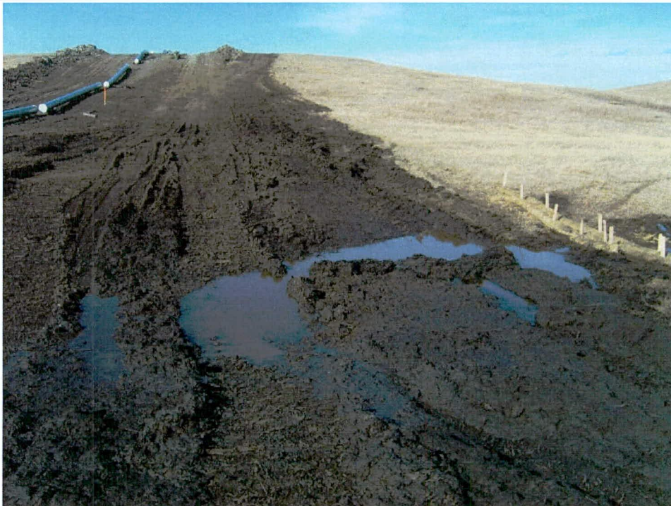
Photo 6 – Rutting and Recommended Placement of Timber Mats
