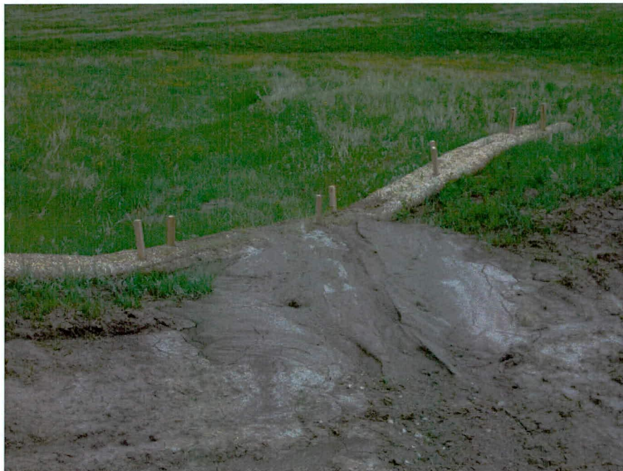
Photo 10 – Erosion Control Repair
