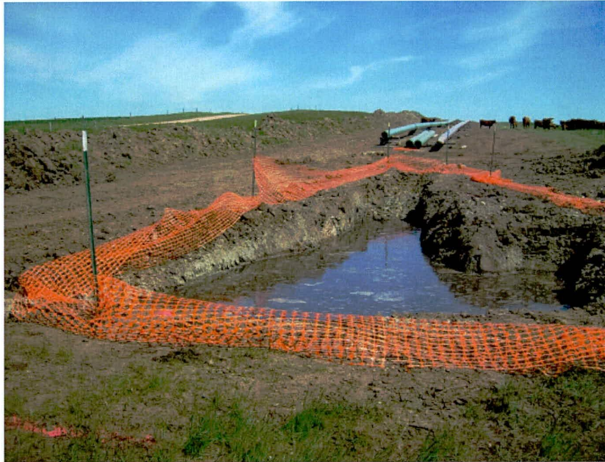
Photo 9 – Construction Fence Repair
