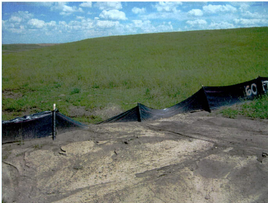
Photo 8 – Silt Fence Repair
