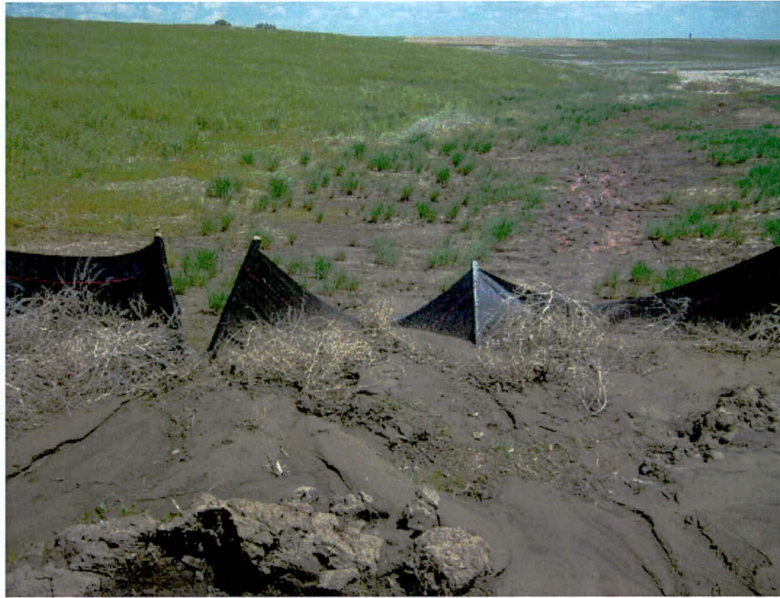
Photo 7 – Silt Fence Repair
