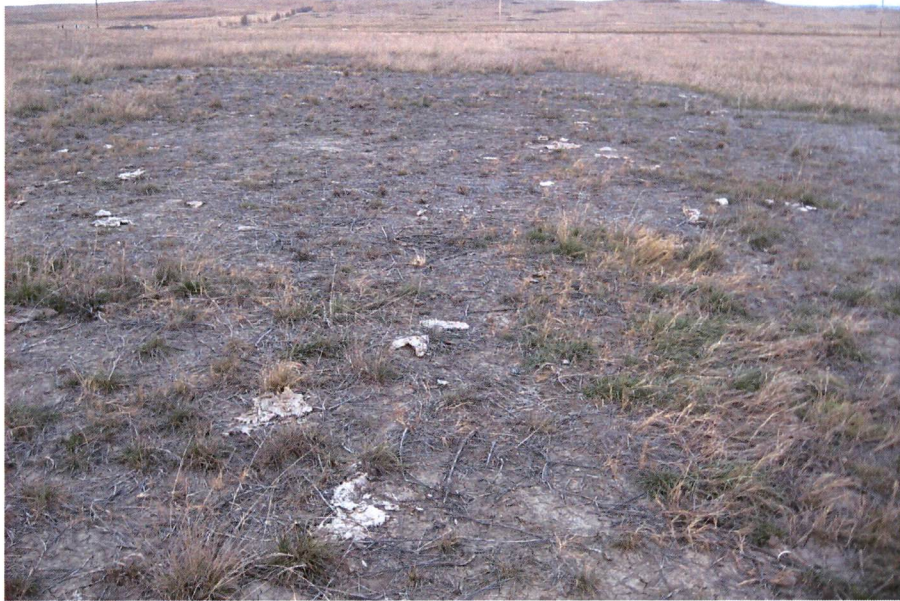
Photo 16 – Approx. Station 160+00. View of revegetation less than 70% south of 7 th Street SW.
