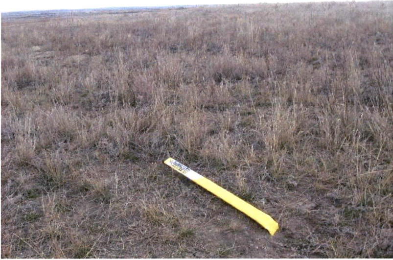
Photo 12 – Approx. Station 820+00. View of fallen pipeline marker.
