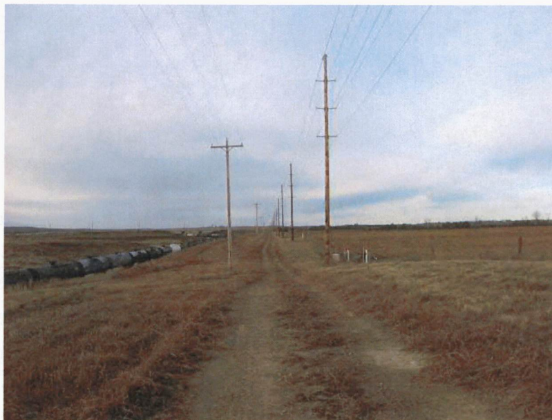
Photo 4 – Approx. Station 2005+00. View of pipeline right of way looking west.
