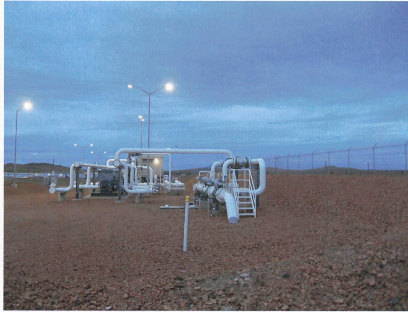
Photo 15 – Station 0+00. View of interconnect location.
