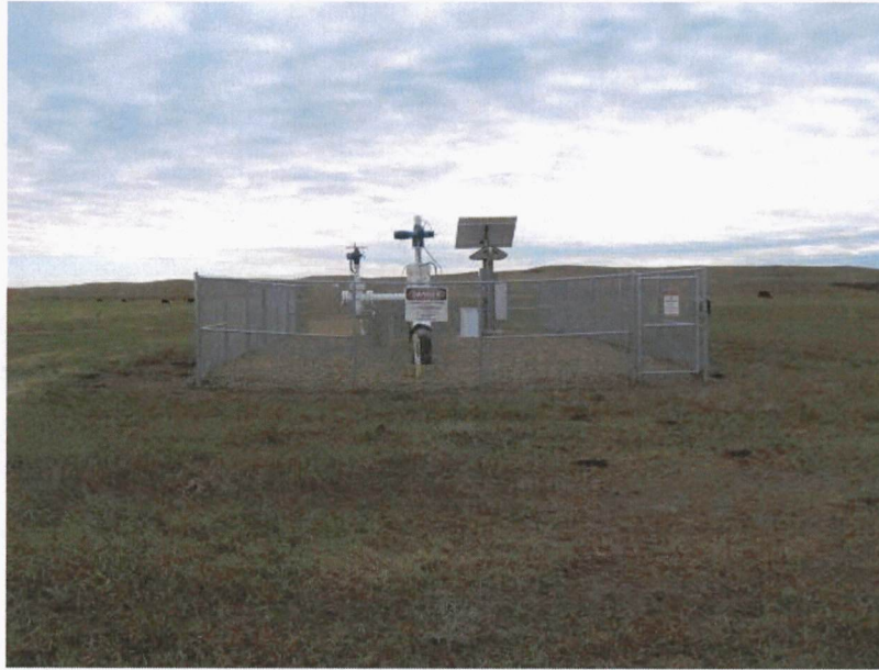
Photo 9 – Approx. Station 1785+00. View of True Oil valve site.
