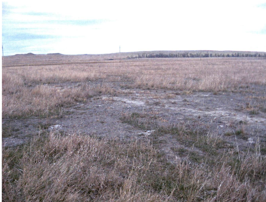
Photo 16 – Approx. Station 160+00. View of revegetation less than 70% south of 7 th Street SW.
