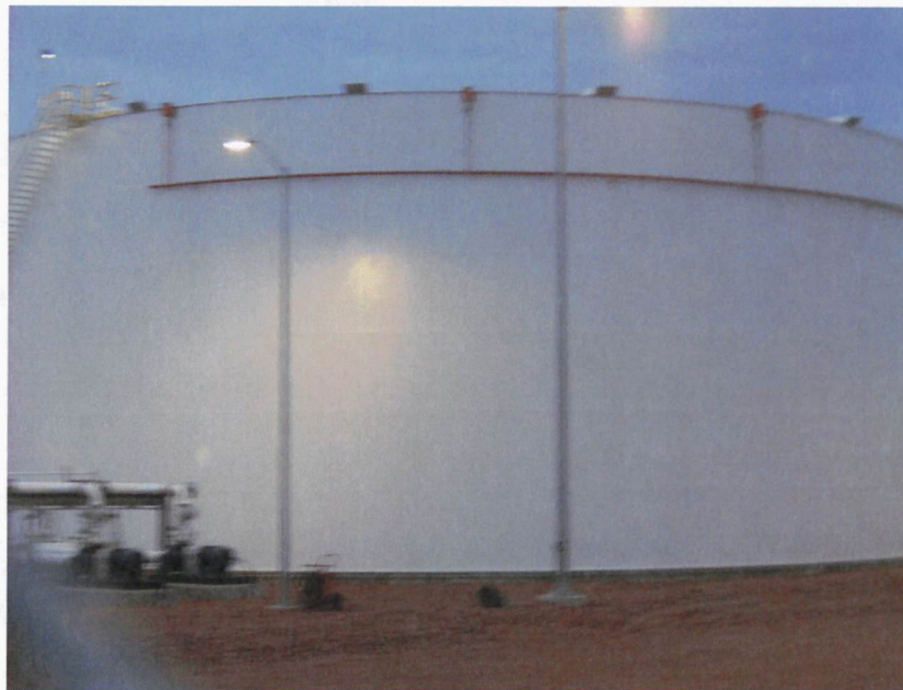
Photo 16 – Station 0+00. View of tank facility at interconnect location.
