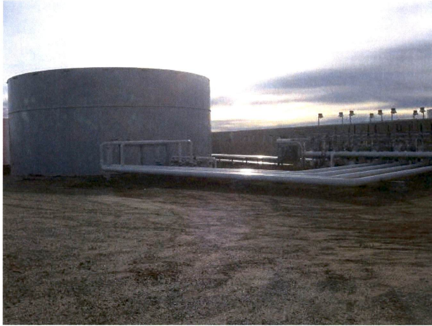
Photo 1 – Station 2016+34. View of interconnect with tank facilities near Dickinson.
