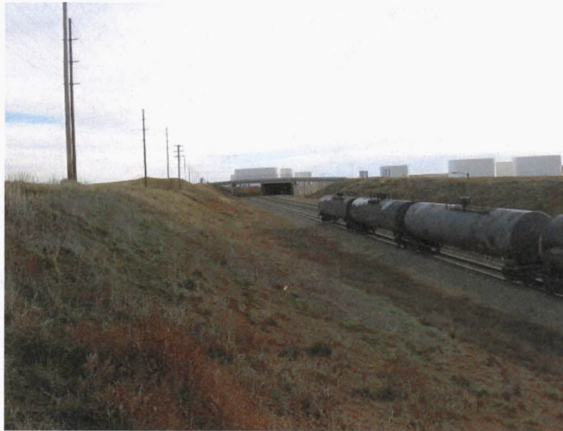
Photo 3 – Approx. Station 2010+00. View of pipeline right of way adjacent to railroad looking east.
