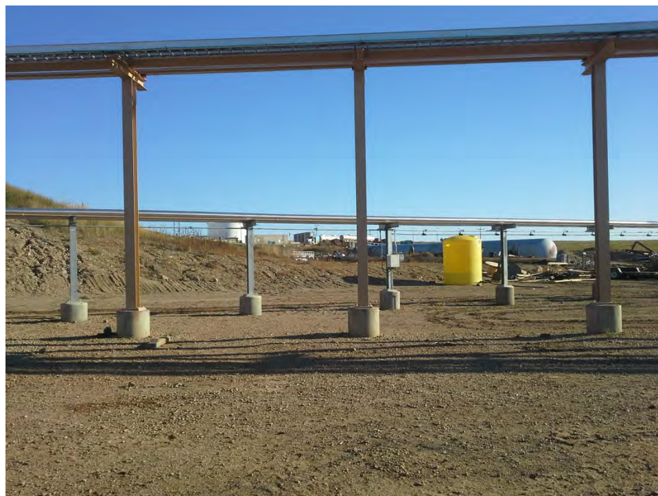
Photo 2. View of condensate storage area facing northeast.
