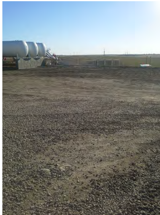
Photo 3. View of proposed compression expansion area facing north.
