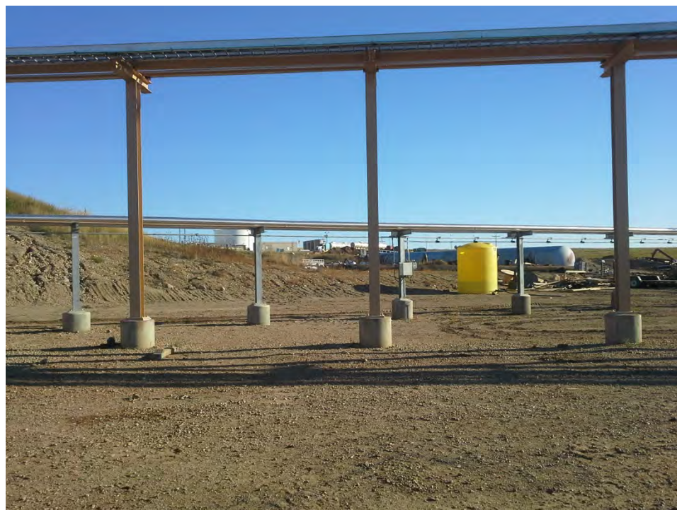
Photo 2. View of condensate storage area facing northeast.
