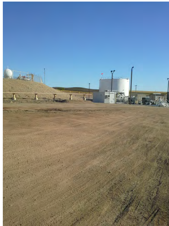
Photo 4. View of east side of proposed compression expansion area facing north.
