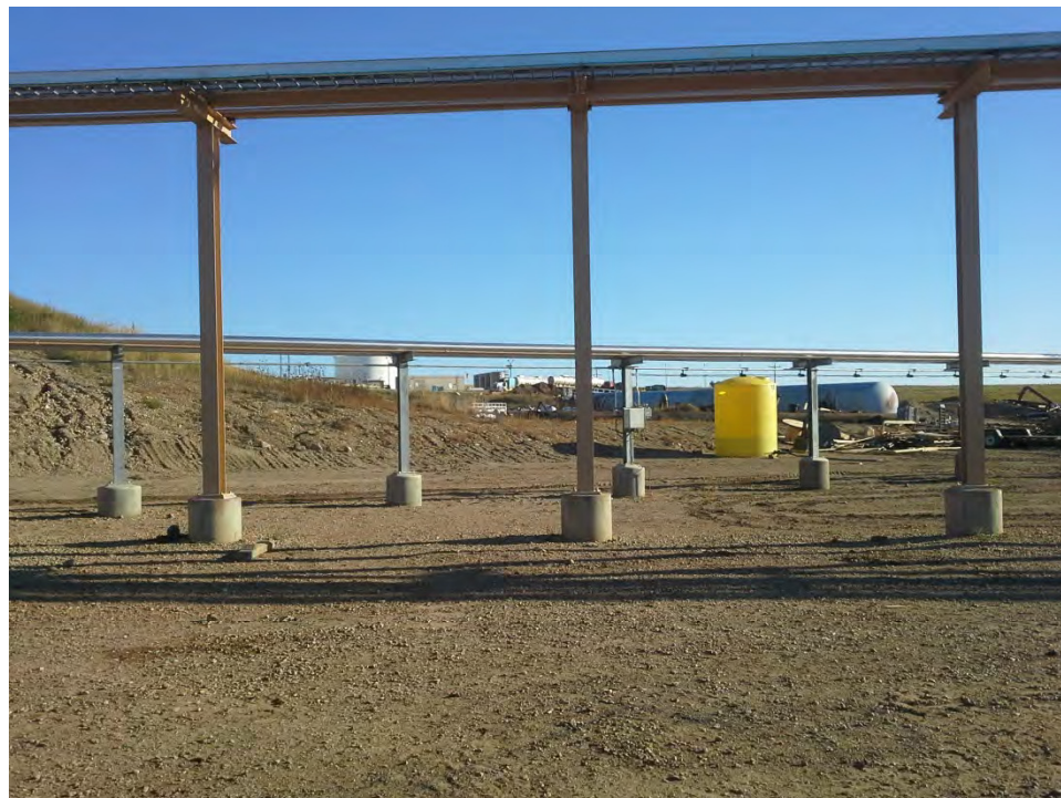
Photo 2. View of condensate storage area facing northeast.
