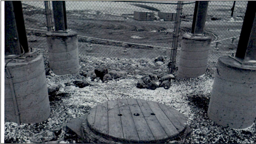
Photo 7: Rip rapped drop that receives runoff from construction area.
