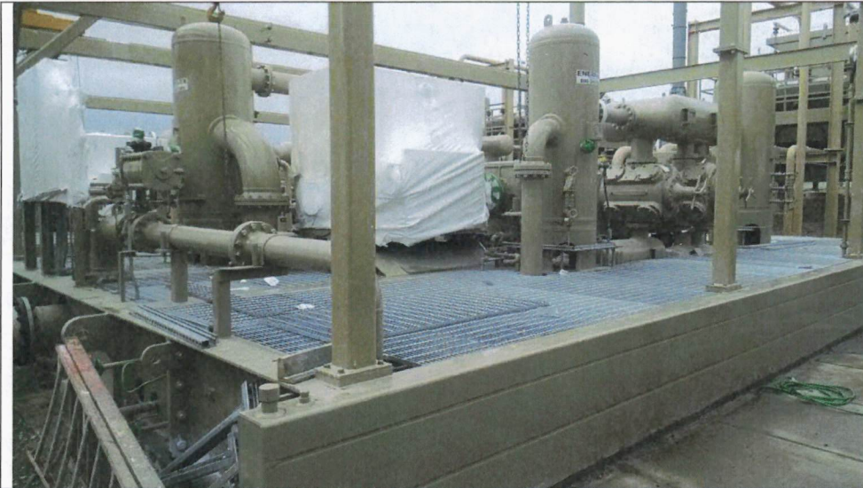
Photo 1: Compressors being installed.
