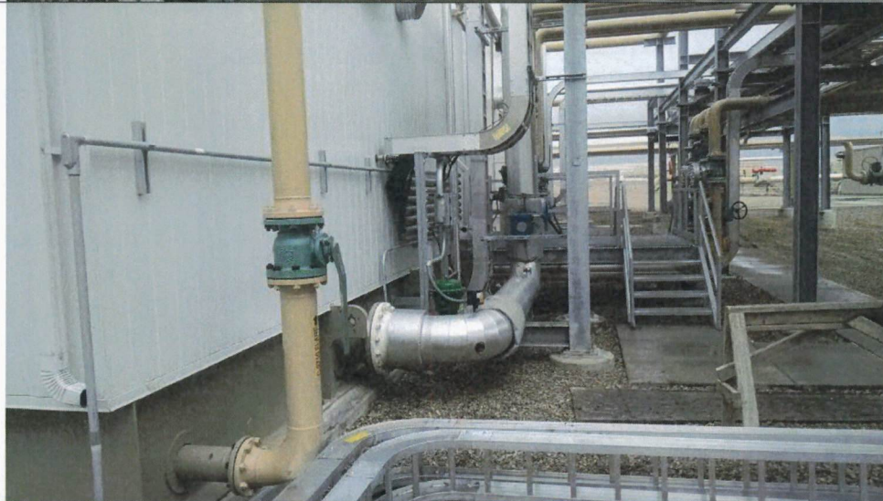
Photo 2: Adjacent existing compressor building
