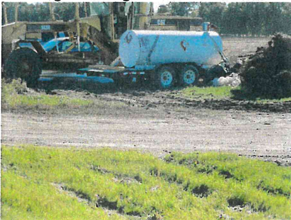
NE Drive Entrance Photo 5 Looking S Constructed Conditions
