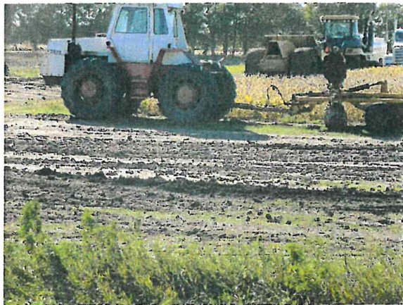
Photo 21 Access Drive to Stock Pile Area Requires revegetation after Construction
