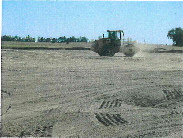
Photo 13 Site Compaction South PL Looking South
