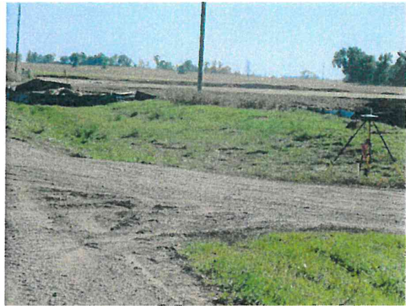
NE Drive Entrance Photo 4 Looking SW Constructed Conditions
