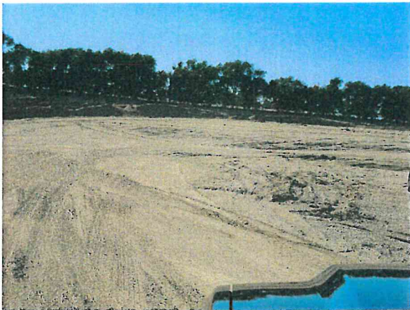
Photo 19 Site Compaction Looking W from S Drive
