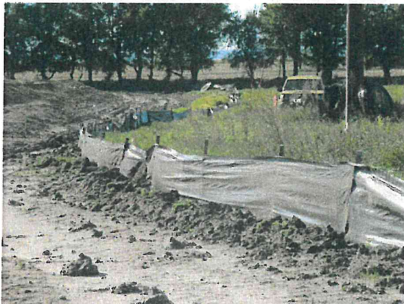
Photo 15 North Prop. Line Erosion Control
